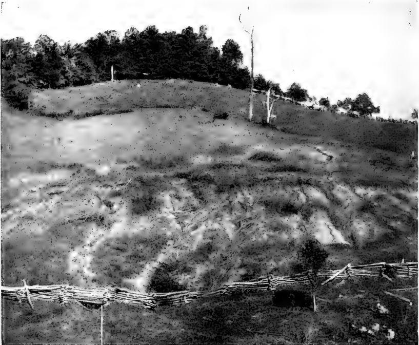
Fig. 250.—Erosion checked by brush dams, Walnut Run, N. C. (Ayres and Ashe, U. S. Geol. Surv.)
