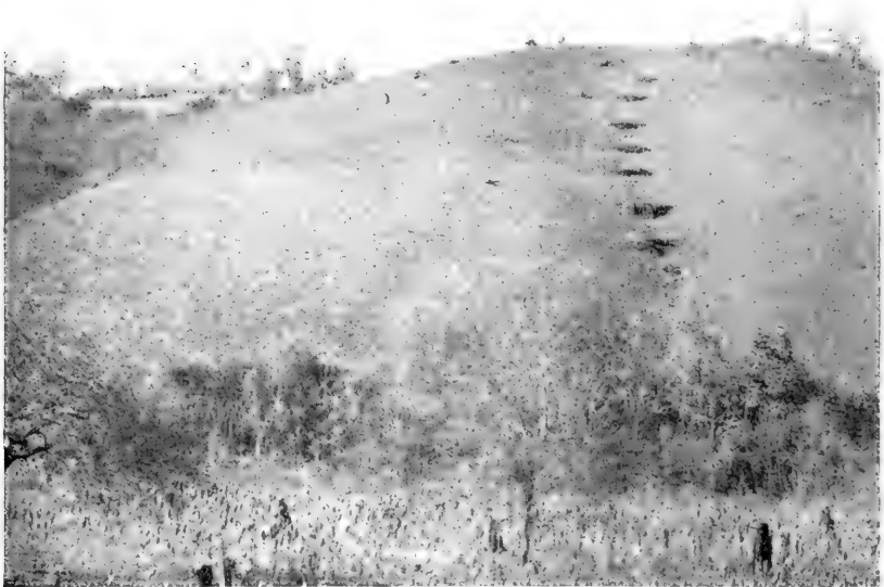
Fig. 249. — Erosion checked by covering gulleys with brush, Longcreek, Va. (Ayres and Ashe, U. S. Geol. Surv.)
