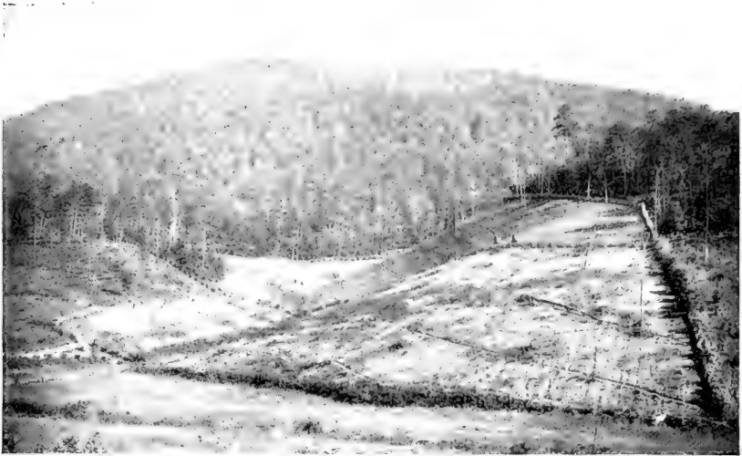
Fig. 248. — Protection against erosion by parallel ditches. (Ayres and Ashe, U. S. Geol. Surv.)
