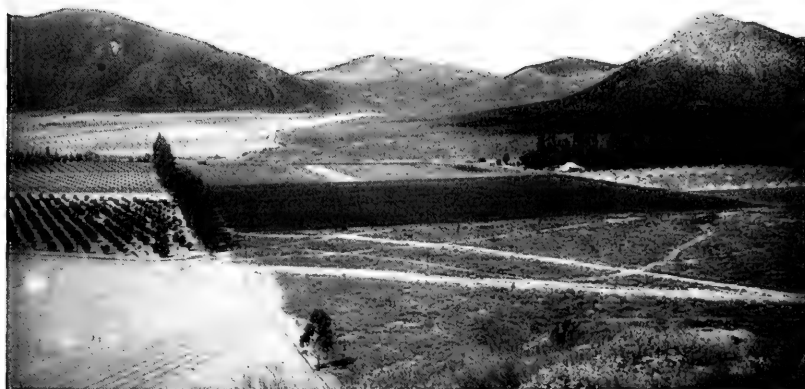
Fig. 46. — West Riverside district, California, representing typical relations of mountains and bordering alluvial plains, valley of southern California. (Mendenhall, U. S. Geol. Surv.)
