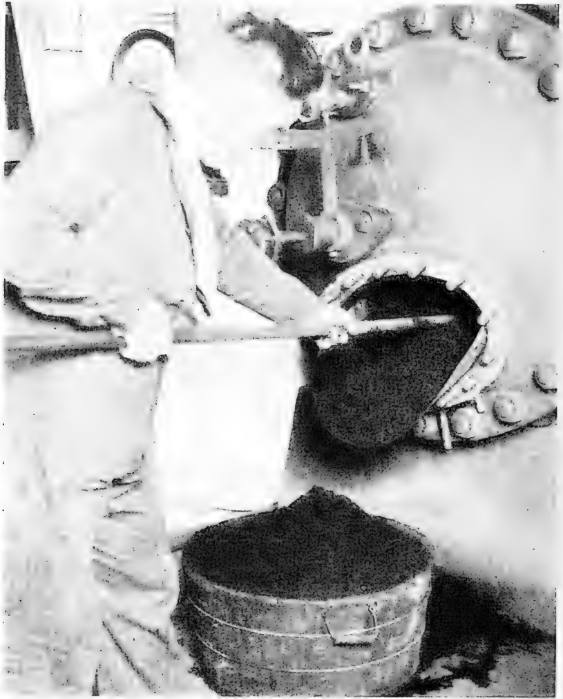
The first step in the manufacture of cattle food from sawdust is to cook the sawdust with dilute acid in a steam-pressure cylinder. This converts a part of the wood into sugars and renders the remainder more digestible. Hydrolyzed sawdust is being successfully fed to cattle as a considerable part of their concentrate ration.
