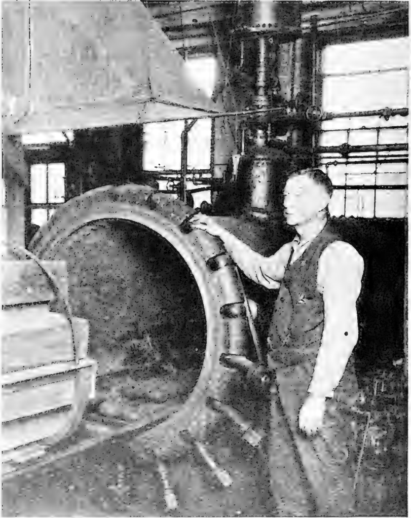
The life of railroad ties treated with preservatives is often double that of untreated ties. The illustration shows some red-oak ties about to undergo an experimental treatment with creosote in the pressure cylinder. Afterwards they will be placed in actual service in one of the test tracks maintained by the railroads in cooperation with the Laboratory
