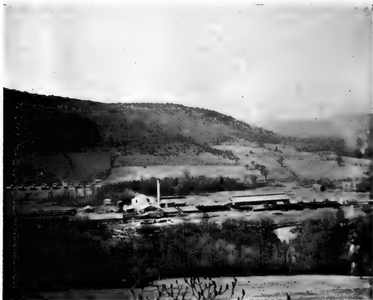
FIG. 56.—General view of hardwood distillation plant at Betula, Pennsylvania. On the left is the wood yard, in the center the oven house and still house and on the right, the charcoal storage warehouse. Immediately to the right of the oven house are the two sets of cooling ovens.
