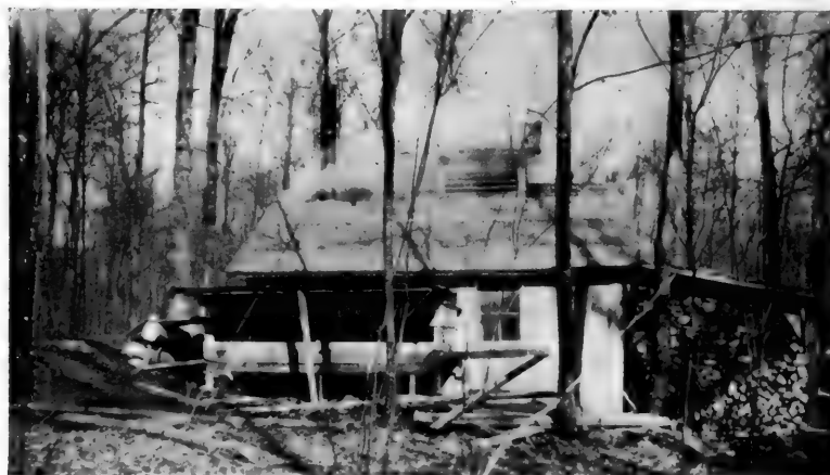
FIG. 103.—A typical sugar house in the "sugar bush." A large pile of dry wood is available for heating the evaporator under the shed at the right.
