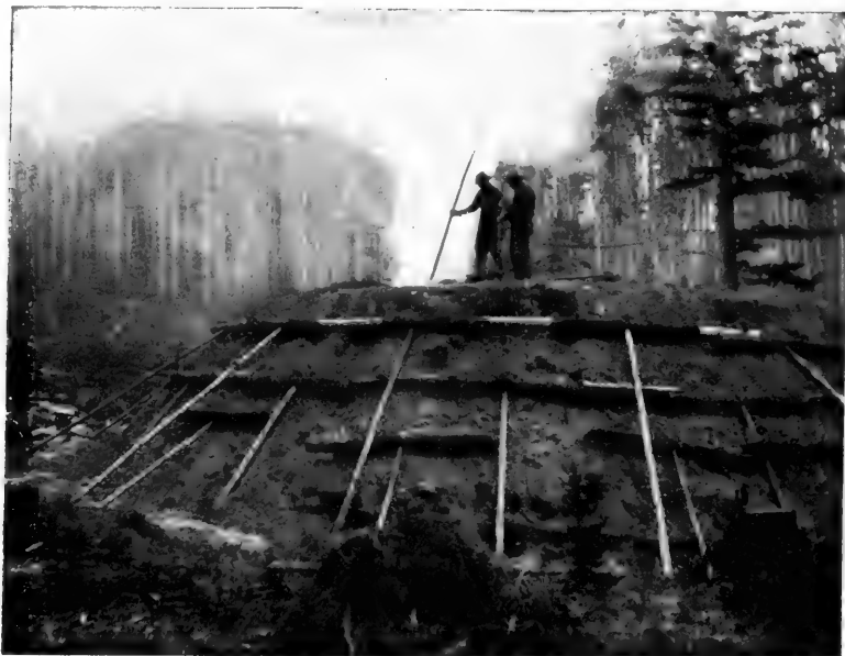
FIG. 64.—A charcoal pit in the process of burning. An "explosion" has occurred and the burners are determining the extent of the cavity. The latter is filled with small pieces of wood which are held in readiness for this purpose. The framework in the exterior is used to hold the dirt in place. Photograph taken in Deerlodge National Forest, Montana. The wood used is lodgepole pine ( Pinus murrayana ).
