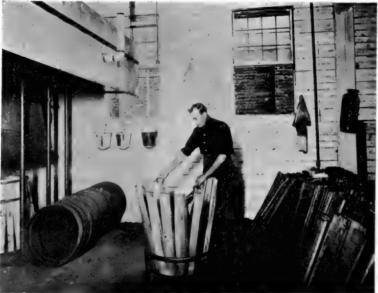
FIG. 32.—First step in assembling a barrel.
