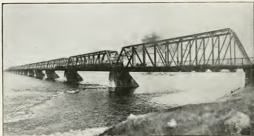
VICTORIA JUBILEE BRIDGE, MONTREAL
