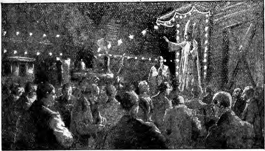
COMPLETING THE LONGEST TUNNEL IN THE WORLD.
