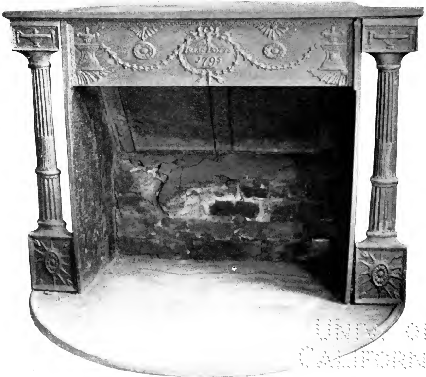
Fireplace in residence of Mr. J. H. Osborne, Summerseat, Morrisville, once Washington's Headquarters. "Isaac Potts, 1795."
