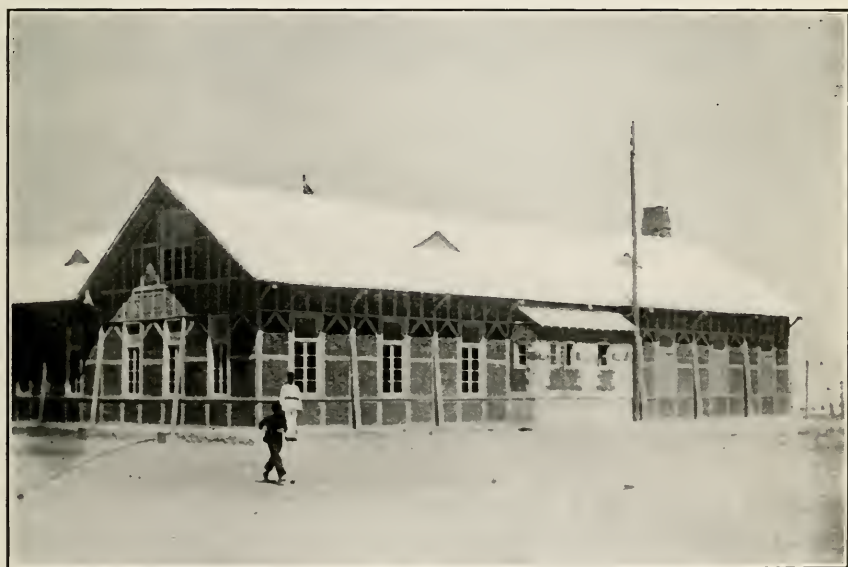
NEW BUILDING FOR SOLDIERS AT ALEXANDRIA (Unlike many others this building is of a semi-permanent nature)
