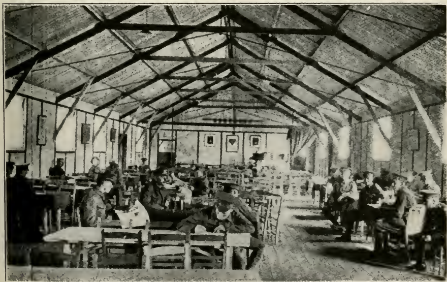
INTERIOR OF THE SAME
