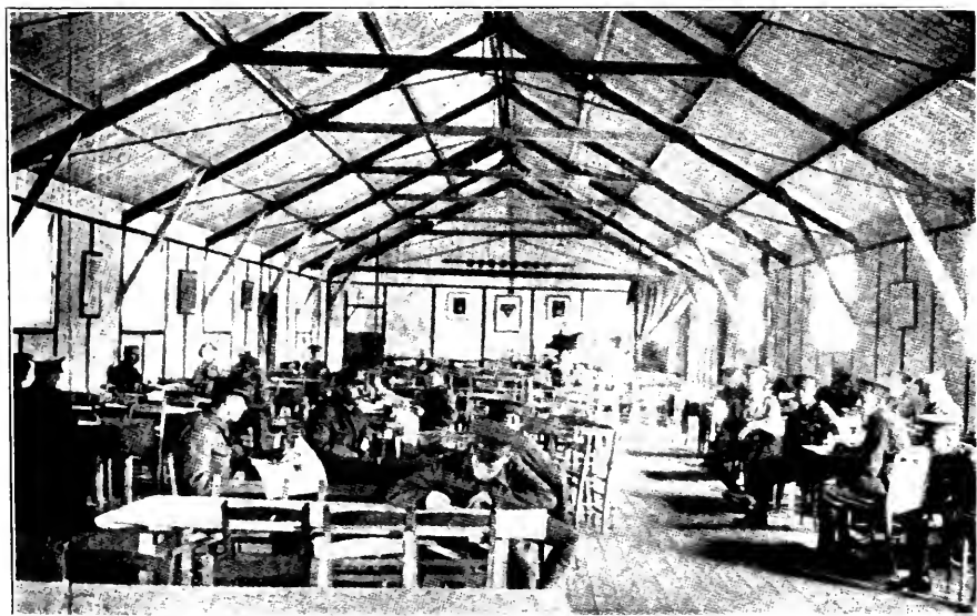
INTERIOR OF THE SAME
