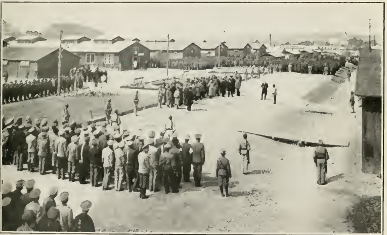
OPENING ASSOCIATION BUILDING (SECOND FROM LEFT) AT WIESELBURG
