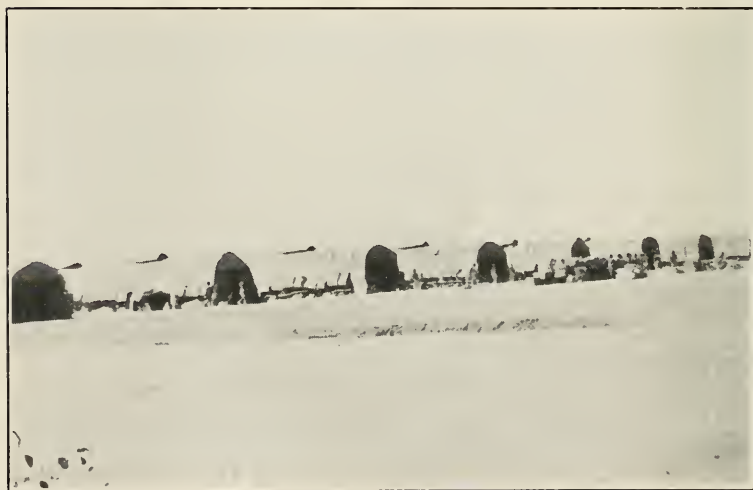
MAT HUTS AT THE BRITISH ARMY BASE IN MESOPOTAMIA One of These is Used by the Association
