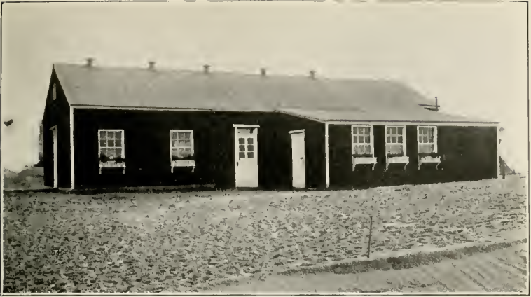
ASSOCIATION BUILDING ON THE ISLE OF JERSEY ERECTED AMID THE DREARY DUNES BY THE PRISONERS THEMSELVES
