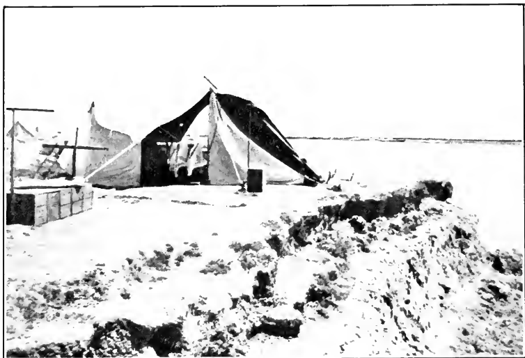
ON THE BANKS OF THE TIGRIS The Post of the Association Four Miles from the Turkish Line
