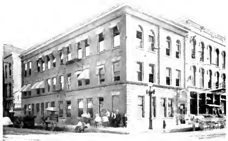
HOME TELEPHONE & TELEGRAPH CO. MAIN OFFICE
