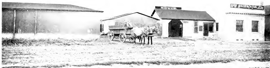
NIEZER AND COMPANY - MAIN OFFICE AND COAL YARDS
