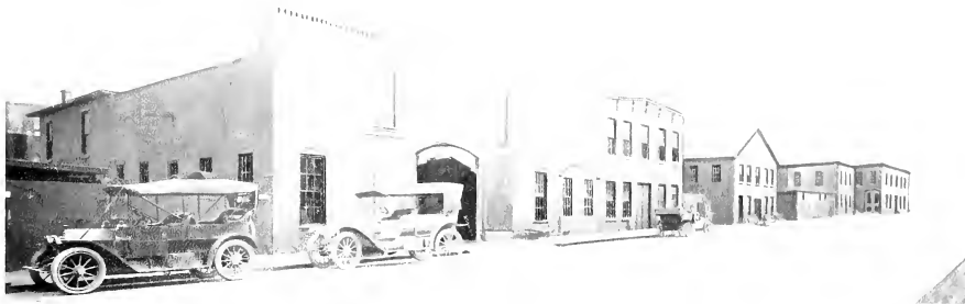
FORT WAYNE FOUNDRY AND MACHINE COMPANY (See Page 1121)
