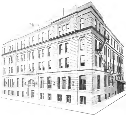
MOSSMAN, YARNELLE AND COMPANY BUILDING
