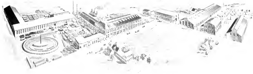
WESTERN GAS CONSTRUCTION CO.
