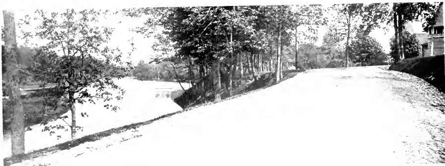
VIEW IN ROBINSON PARK
