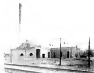
PUMPING STATION NUMBER ONE
