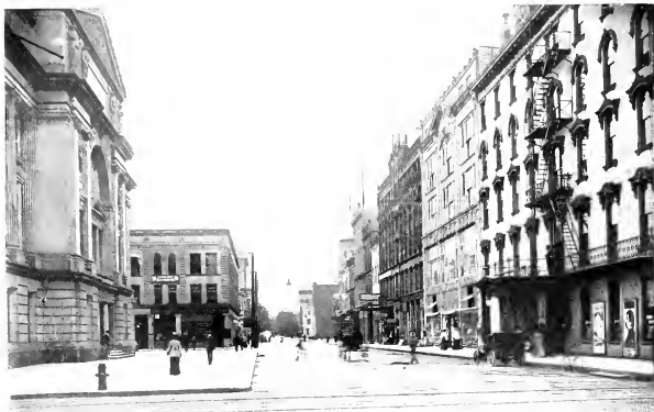
BERRY STREET, LOOKING EAST FROM CALHOUN STREET
