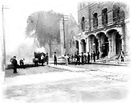
BARBER ASPHALT COMPANY'S MEN LAYING TRINIDAD PITCH LAKE ASPHALT ON A FORT WAYNE STREET
