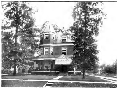
RESIDENCE OF FRANK V. CULBERTSON
