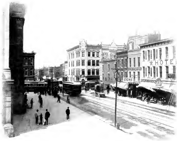
CITY TERMINAL OF URBAN AND INTERURBAN STREET CAR LINES
