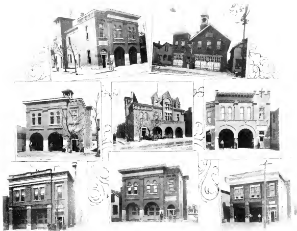
GROUP OF FIRE DEPARTMENT BUILDINGS
