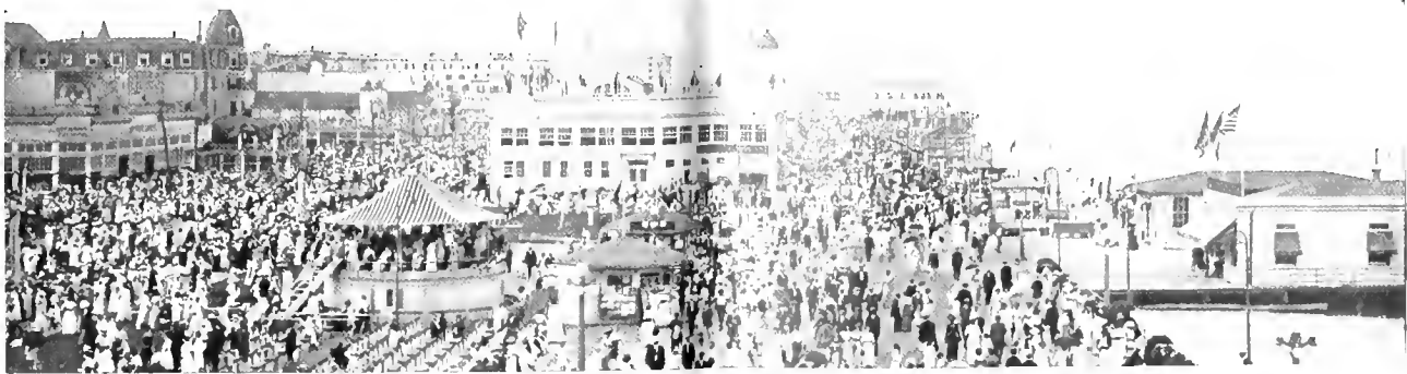
ASBURY PARK BOARDWALK
