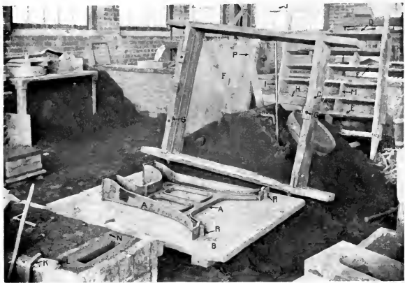
FIG. 17.—PATTERN OF LATHE-BED LEGS LAID ON MOLD-BOARD READY FOR FLOOR MOLDING.
