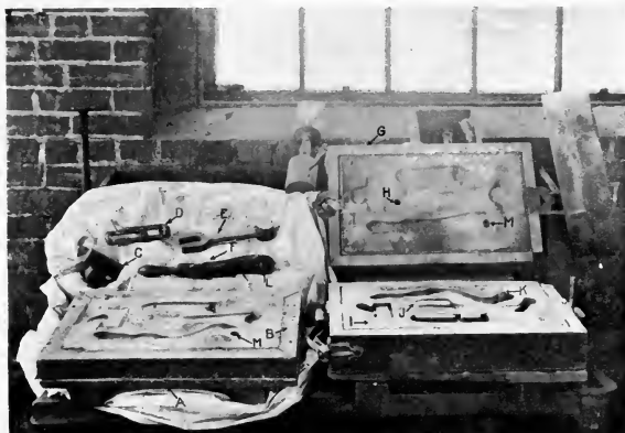
FIG. 9.—MOLDING IRREGULARLY SHAPED PATTERNS WITH A GREEN-SAND MATCH.
