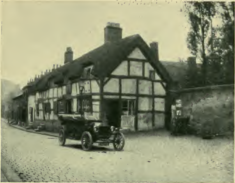
HALF-TIMBERED COTTAGES IN DARKNESS LANE
