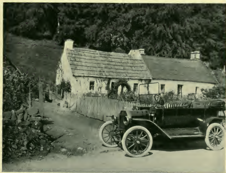
A HIGHLAND COTTAGE WITH ONE THATCHED CHIMNEY
