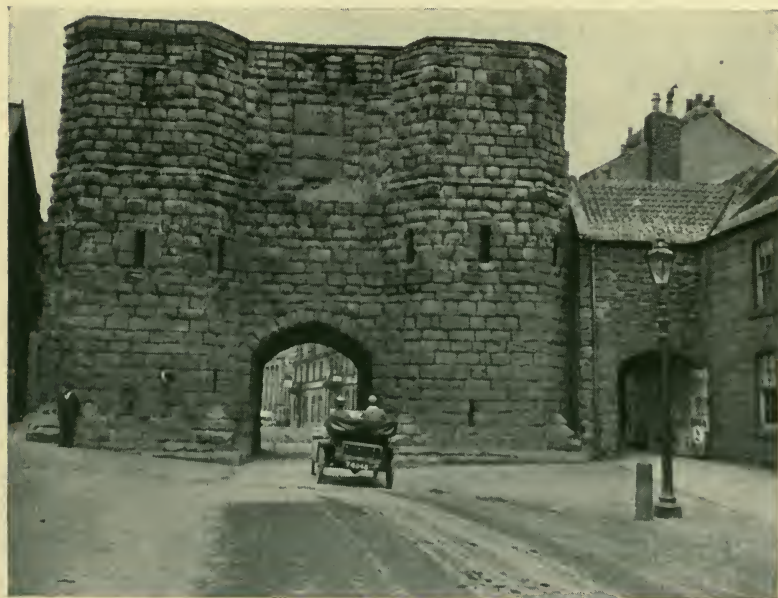
THE TOWN-GATE OF DISMAL ALNWICK
