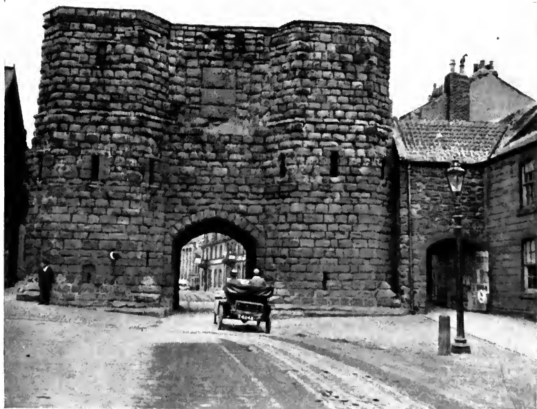
THE TOWN-GATE OF DISMAL ALNWICK
