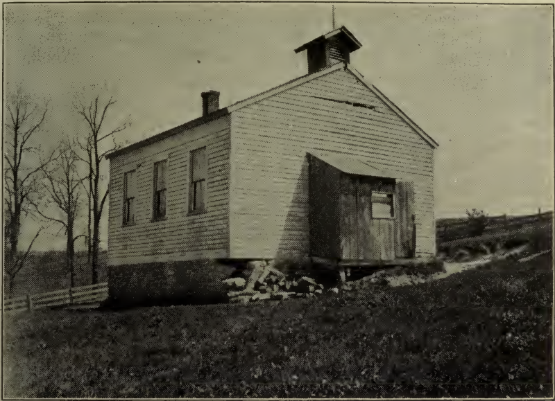
One of the Buildings Condemned
