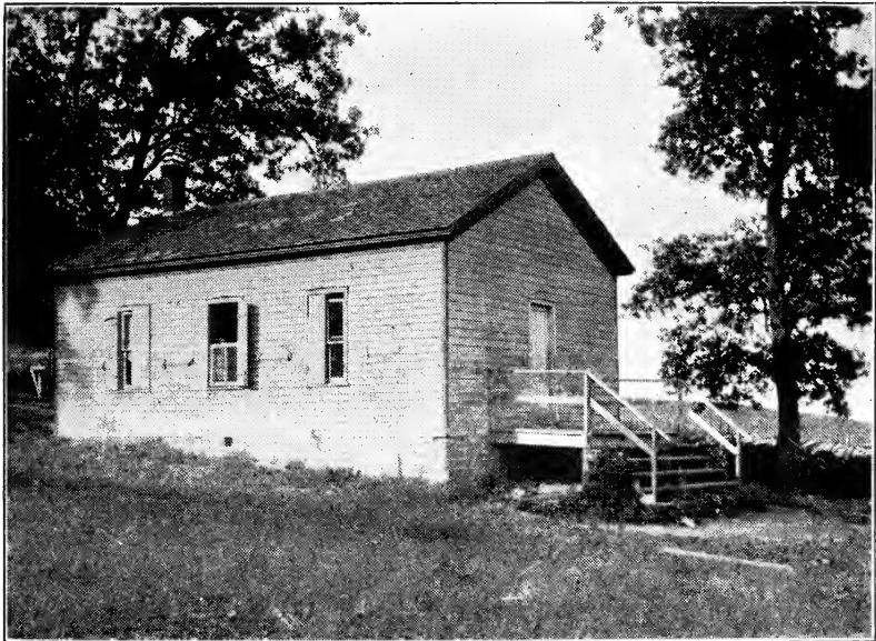
Another Schoolhouse That Has Been Condemned
