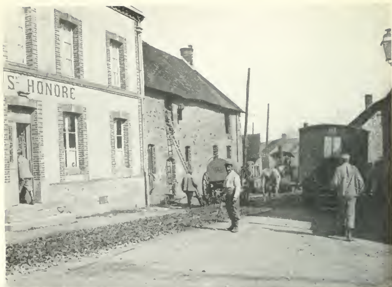
Repairing Road in a Marne Village.
