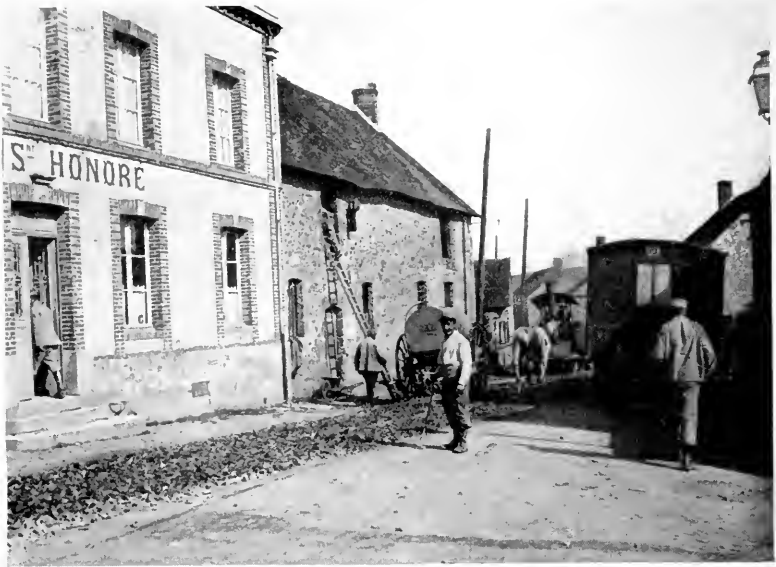
Repairing Road in a Marne Village.
