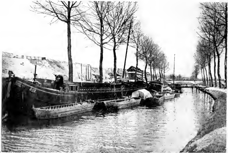
Barges on the Meuse Canal Near Rheims—1919.
