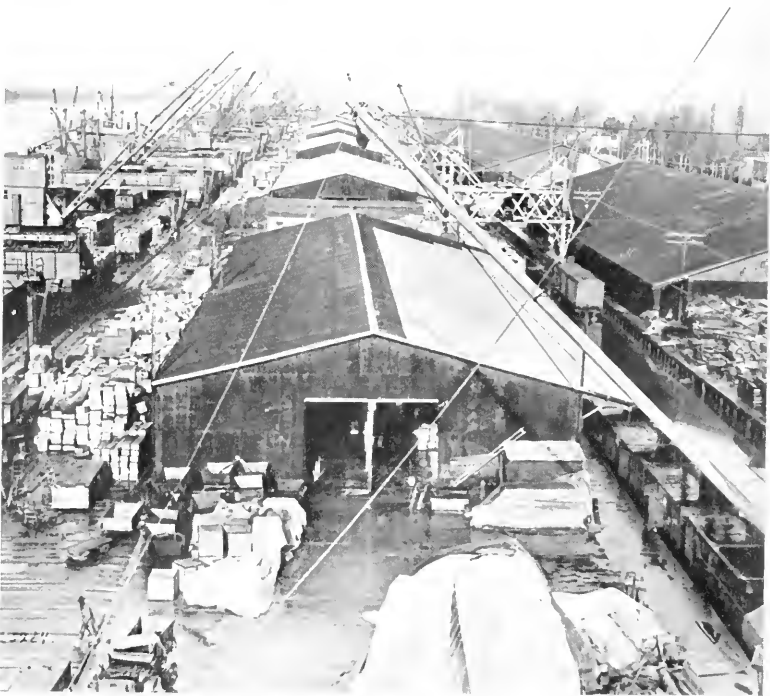
Docking and Warehousing Facilities Near Bordeaux.
