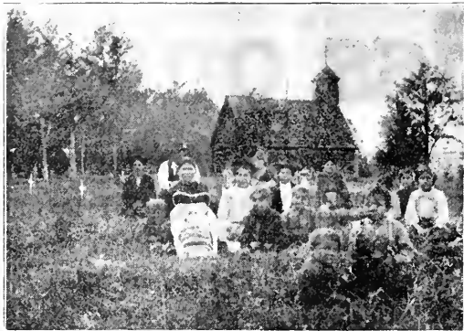
Chapel at Mouth of Yellow River destroyed by fire, 1915.
