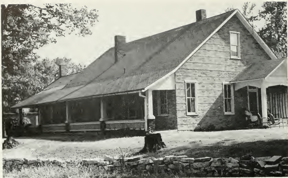
EARLIER FAULKS HOUSE CALLED HALF-WAY HOUSE (LINCOLN IS REPUTED TO HAVE STOPPED HERE)
