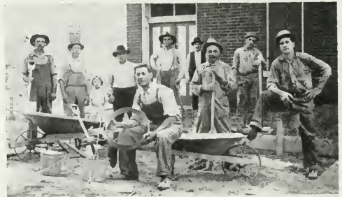
POURING CONCRETE AT THE OLD CITY HALL
