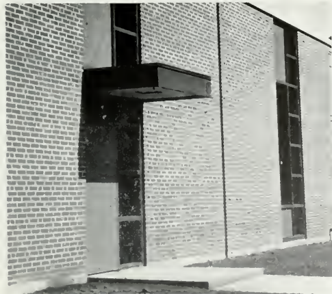
NEW BELL TELEPHONE EXCHANGE UNDER CONSTRUCTION
