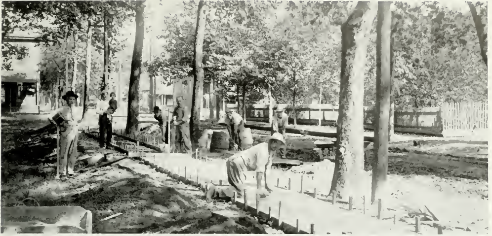
SIDEWALK CONSTRUCTION AROUND THE PARK
