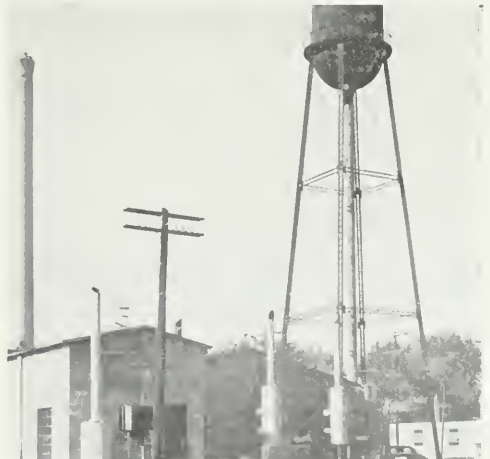
FREEBURG MUNICIPAL LIGHT PLANT WITH NEW FREEBURG VOLUNTEER FIRE DEPT.
