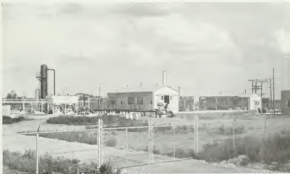
NEW GAS STORAGE FACILITIES - ILLINOIS POWER COMPANY
