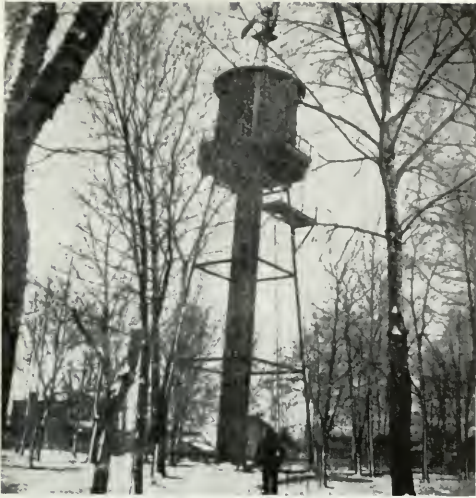
WELL IN PARK WITH FIRST WATER TOWER AND WINDMILL. FIRST PICTURE TAKEN BY RUSSELL HAMILL, MARCH 5, 1899.
