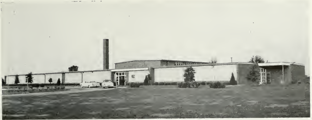
PRESENT FREEBURG ELEMENTARY SCHOOL
