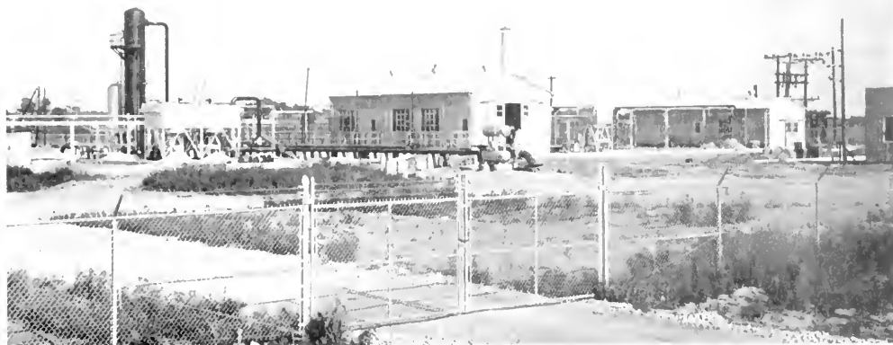
NEW GAS STORAGE FACILITIES - ILLINOIS POWER COMPANY
