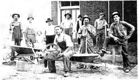
POURING CONCRETE AT THE OLD CITY HALL
