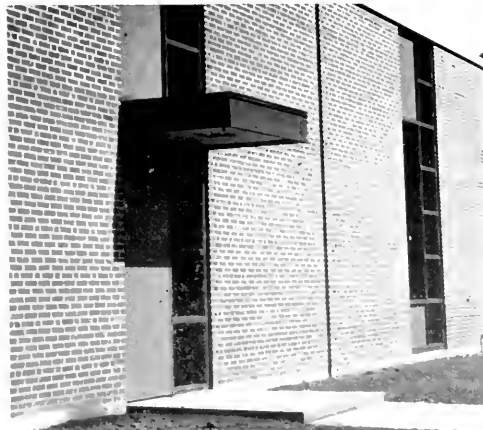
NEW BELL TELEPHONE EXCHANGE UNDER CONSTRUCTION
