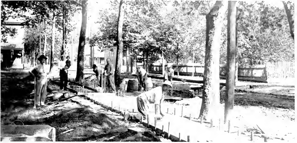
SIDEWALK CONSTRUCTION AROUND THE PARK
