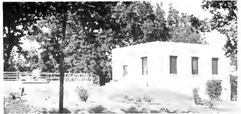
FREEBURG'S NEW WATER FILTRATION PLANT ON SILVER CREEK
