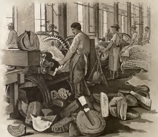
FIRST PROCESS.—GRINDING CRUDE RUBBER.
