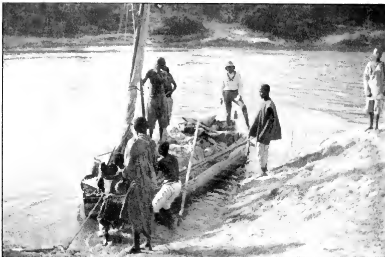
ONE OF THE STEEL BOATS ON THE RIVER YO
