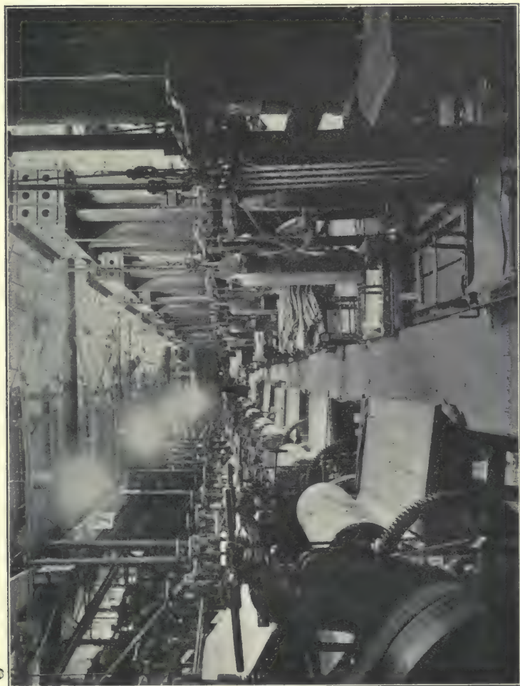
WET MACHINES WHERE THE PULP IS CUT OFF IN SHEETS, THE BROWN CO. To the right are the hydraulic presses for removing moisture from the pulp. The pulp is shipped about seventy per cent moist.
