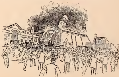
Burning of the Cold Storage Building.
