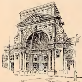
Main Doorway—Electricity Building.
