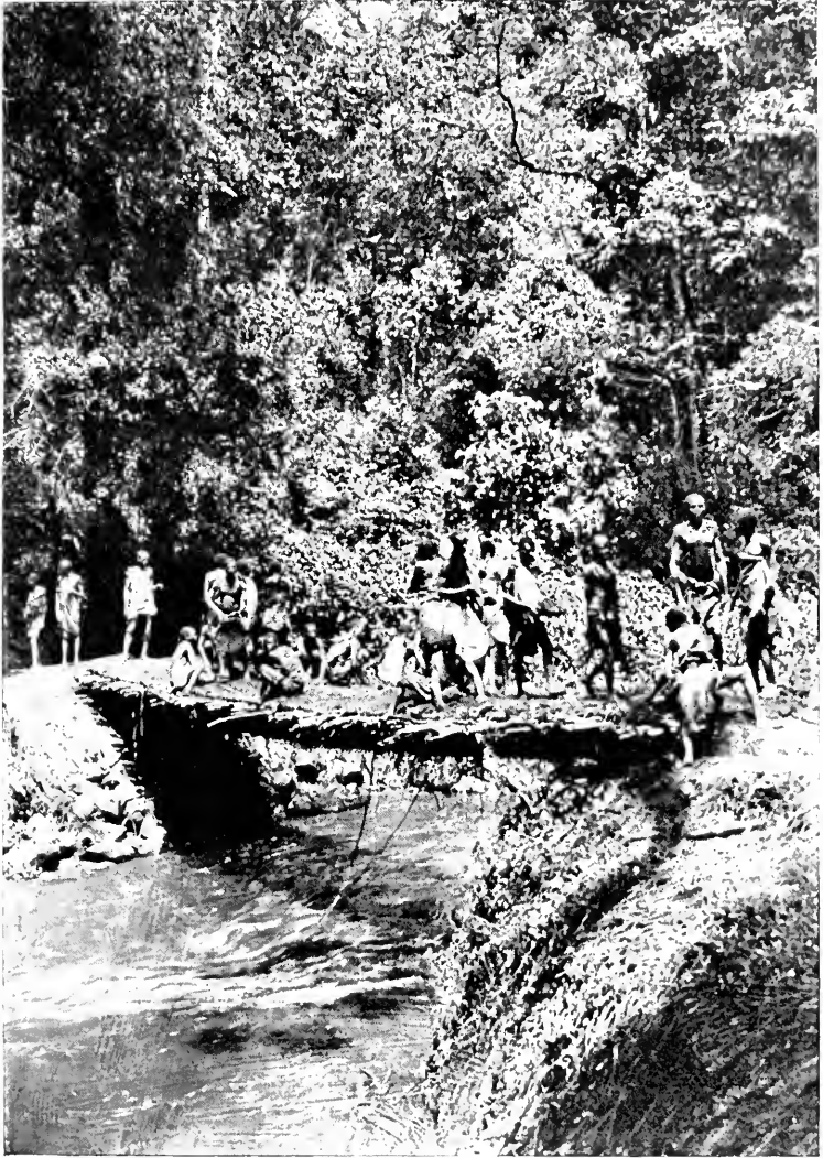
Bridge-Building in Uganda.
