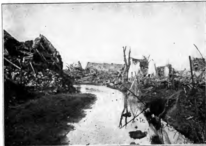
SIDE STREET IN FISMES—WATER BACKING UP FROM THE CHOKED RIVER INTO THE TOWN
