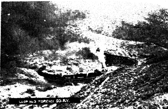
A loop on the Morenci Southern Railroad, the corkscrew road of America. Owned by the Phelps Dodge Copper Company of Morenci
