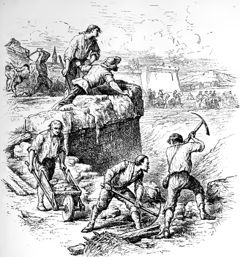
DEMOLISHING THE FORTIFICATIONS. — Page 244.
