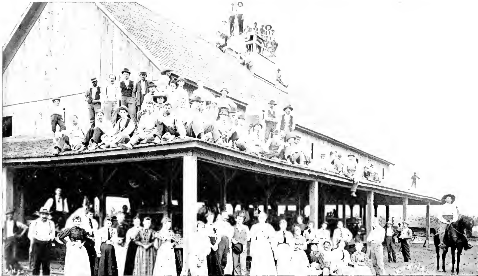
PEACH PACKING HOUSE, NEAR FORT VALLEY, GA.
