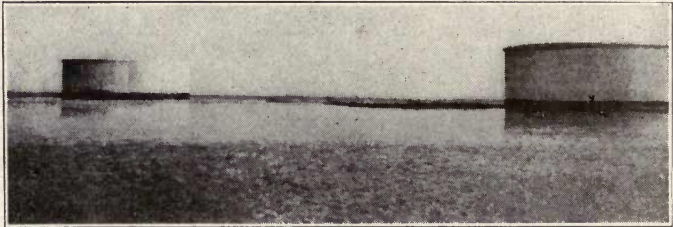
FIG. 28. Concrete Oil Tanks Which Without Damage Withstood a Hurricane and Flood.
