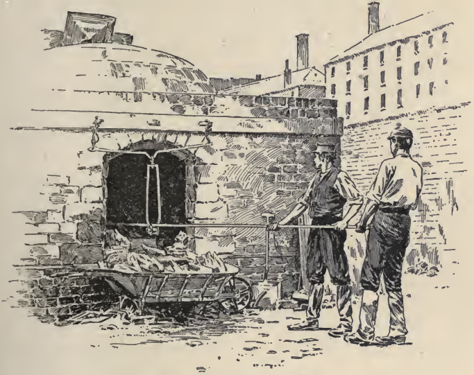
Fig. 9.—Discharging Coke Ovens.
