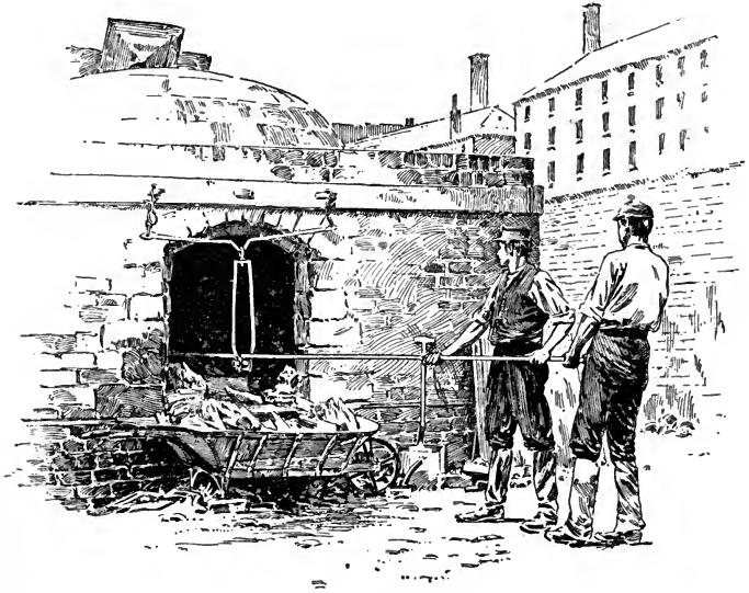
Fig. 9.—Discharging Coke Ovens.
