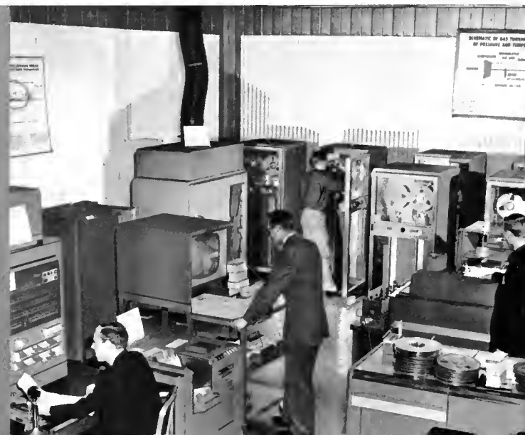
The digital computer room is a busy place.
