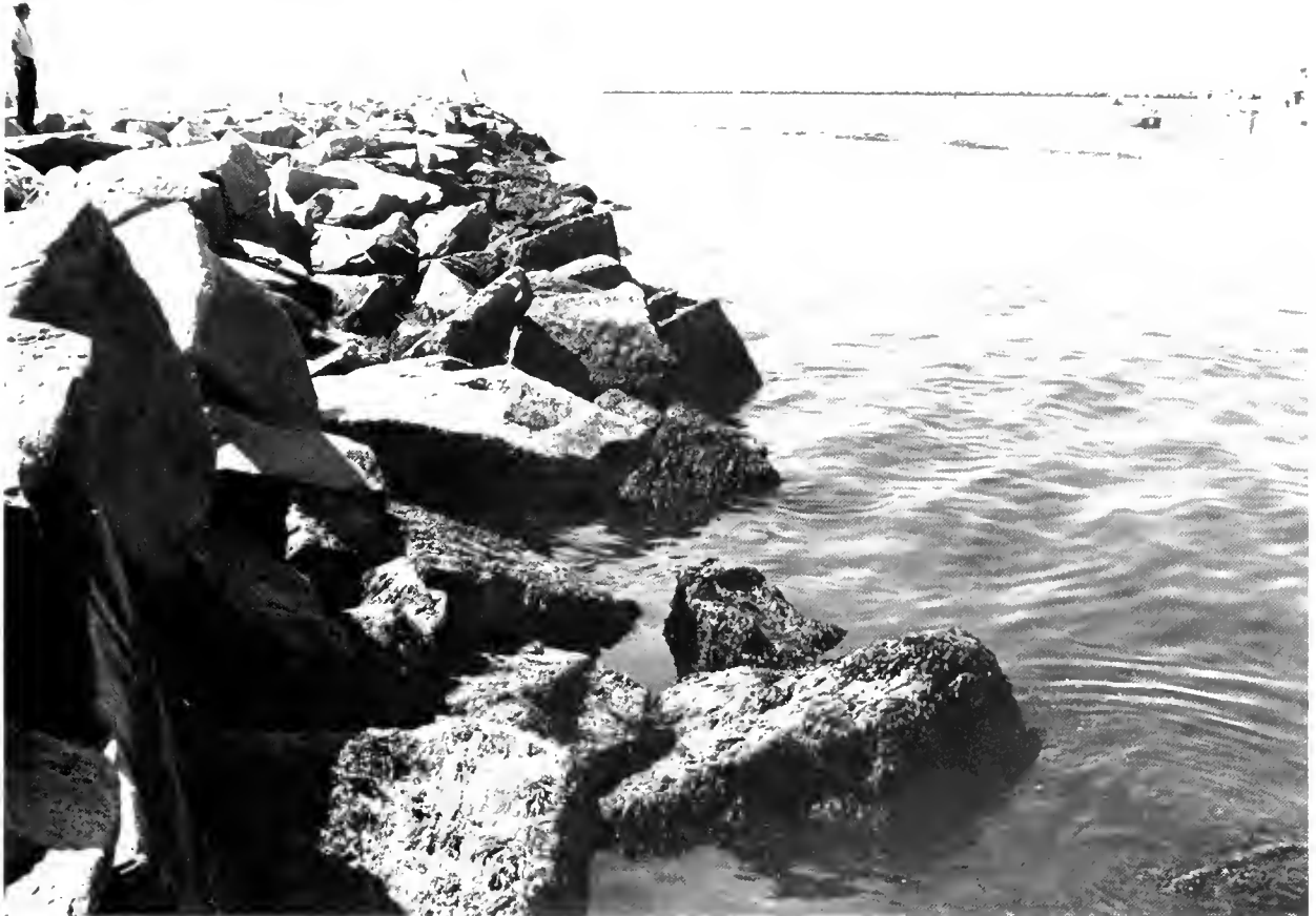
Plate 12. —Two habitats lie at the edge of this manmade breakwater. Classification of upper (lighter) zone: SYSTEM Estuarine, SUBSYSTEM Intertidal, CLASS Rocky Shore, SUBCLASS Rubble, WATER REGIME Irregularly Flooded, WATER CHEMISTRY Euhaline, SPECIAL MODIFIER Artificial. Classification of lower (darker) zone: SYSTEM Estuarine, SUBSYSTEM Intertidal, CLASS Aquatic Bed, SUBCLASS Algal, DOMINANCE TYPE Fucus vesiculosus , WATER REGIME Regularly Flooded, WATER CHEMISTRY Euhaline, SPECIAL MODIFIER Artificial. (Washington County, Rhode Island; July 1977; Photo by F. C. Golet)
