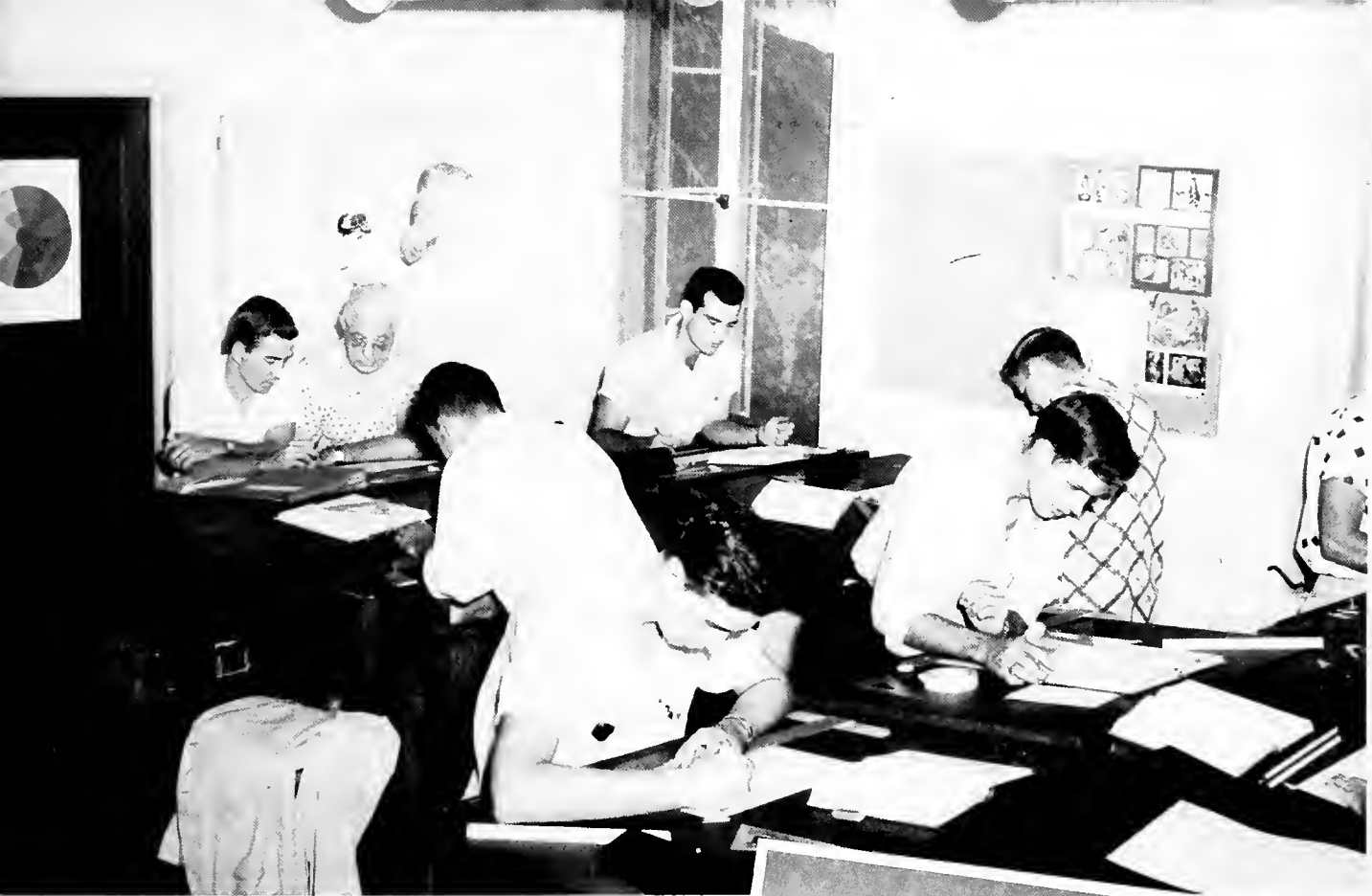
Coats off, sleeves rolled up, as the engineers get down to business.
