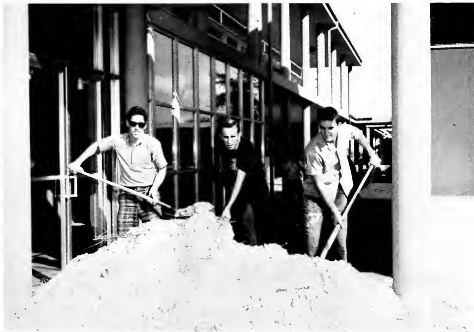
Richard Bernstein, Ken Bucher, and Bruce Mitchell help build a walk by Dean Glynn's office to eliminate a dangerous step down.
