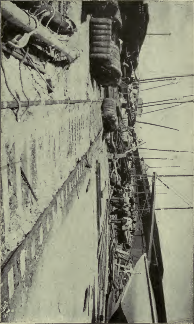
WRECKAGE AT THE COTTON PIERS.
