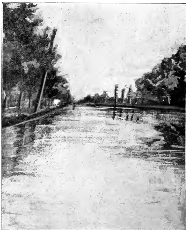
CRAWFORD STREET INUNDATED AND BLOCKED WITH POLES.
