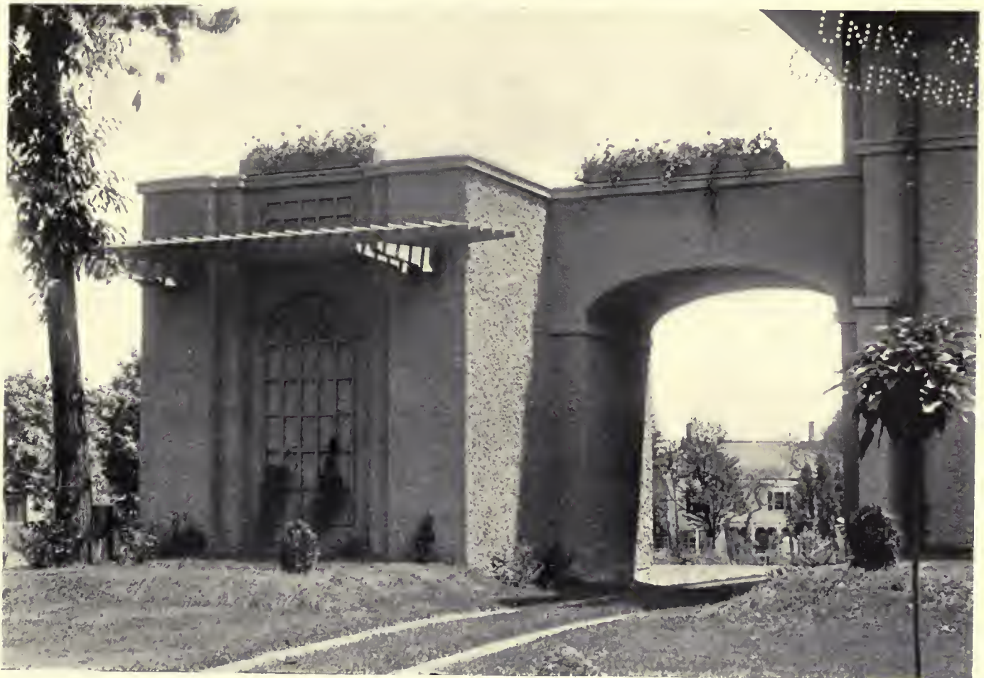
STREET FRONT AND REAR VIEW OF A "ROUGH COAT" GARAGE ON RIDGEWOOD AVENUE, GLENRIDGE, N. J.
