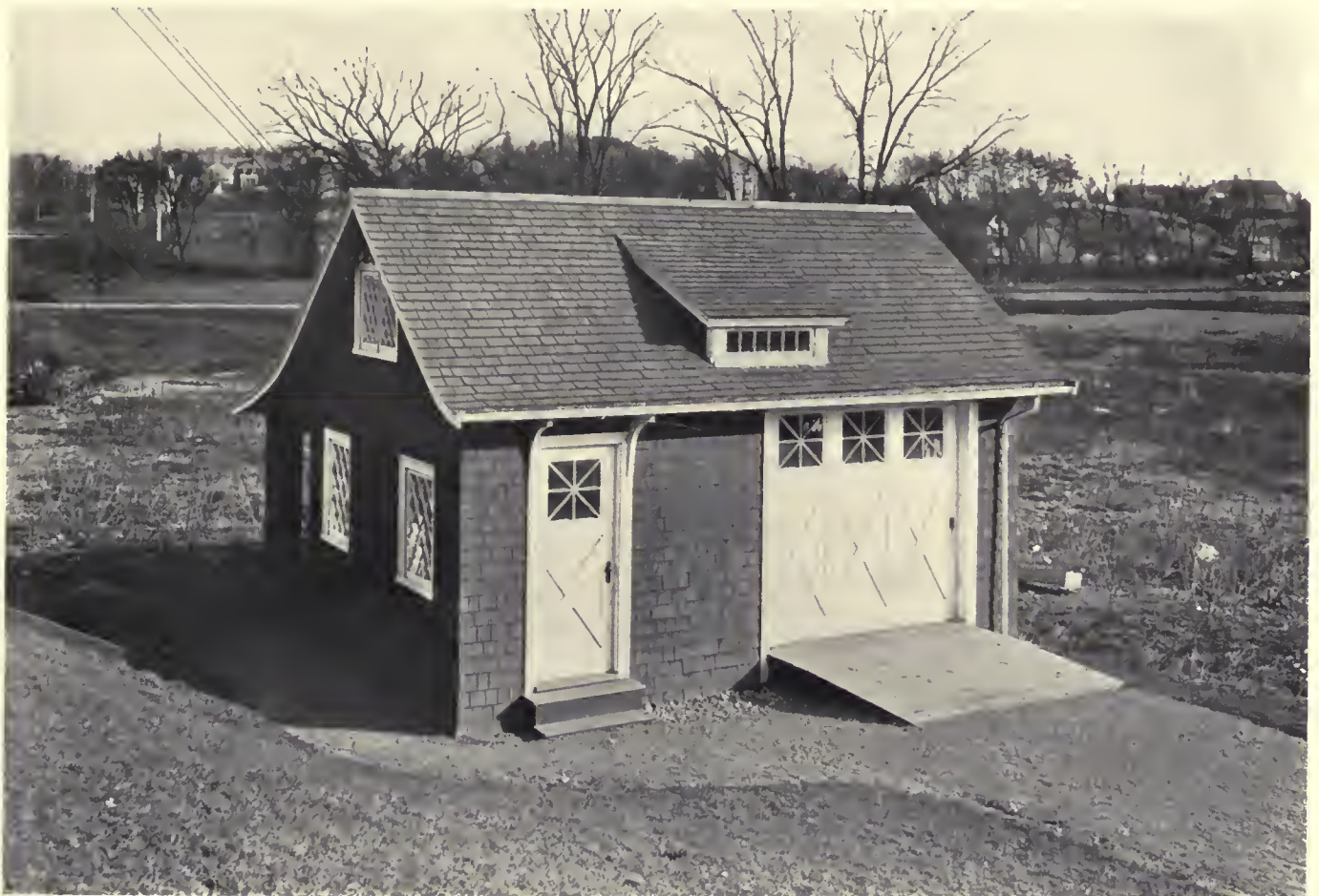
A SHINGLED ONE-CAR GARAGE, WINCHESTER, MASS. Edwin R. Blaikie, Architect
