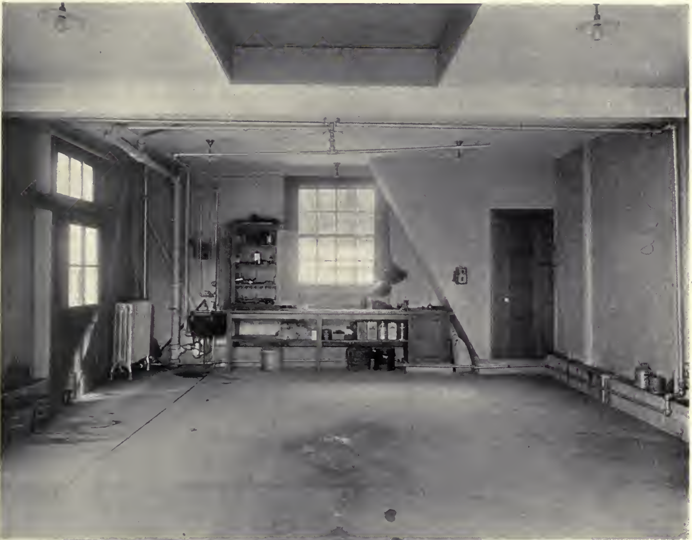
INTERIOR OF GARAGE FOR MR. BERNARD JENNY, JR., BROOKLINE, MASS. Messrs. Kilham & Hopkins, Architects
