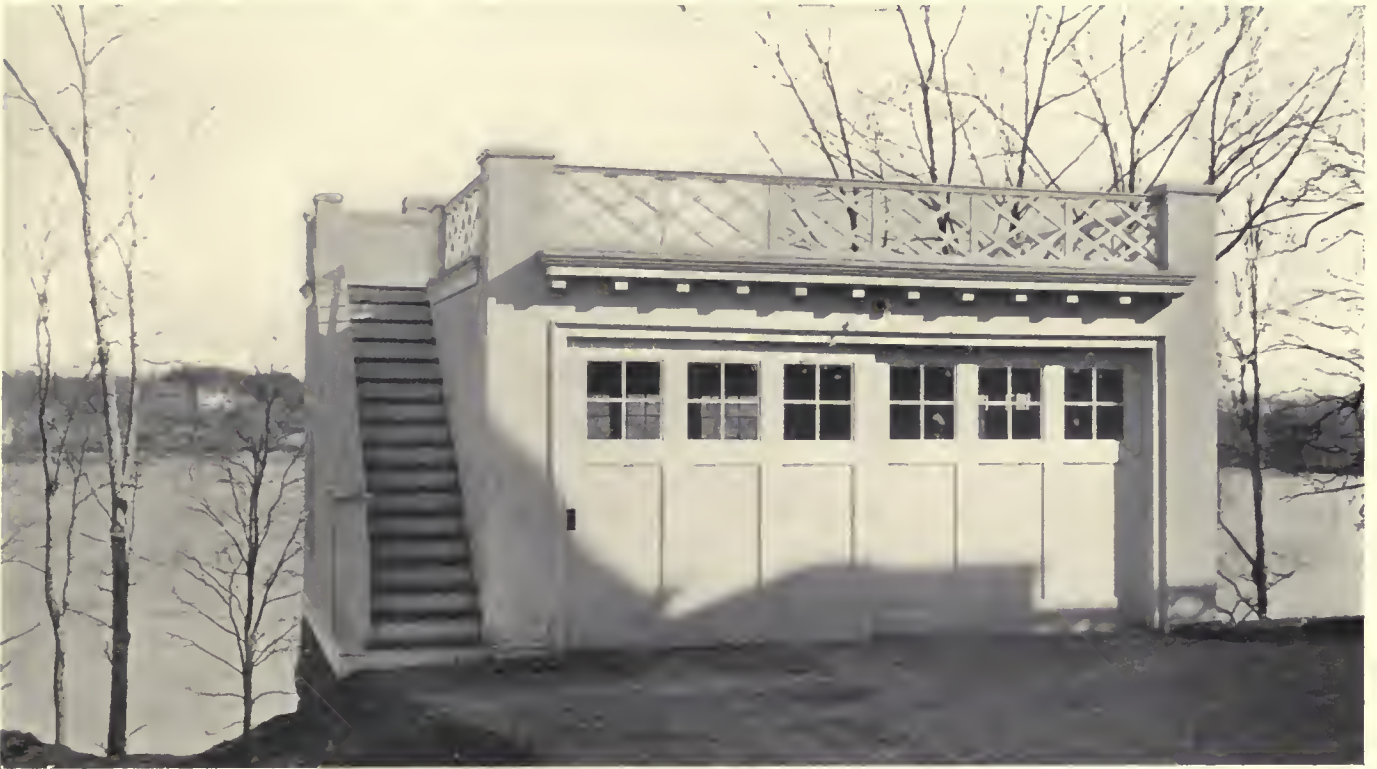
CONCRETE GARAGE OVERLOOKING LAKE NEAR WINCHESTER, MASS.
