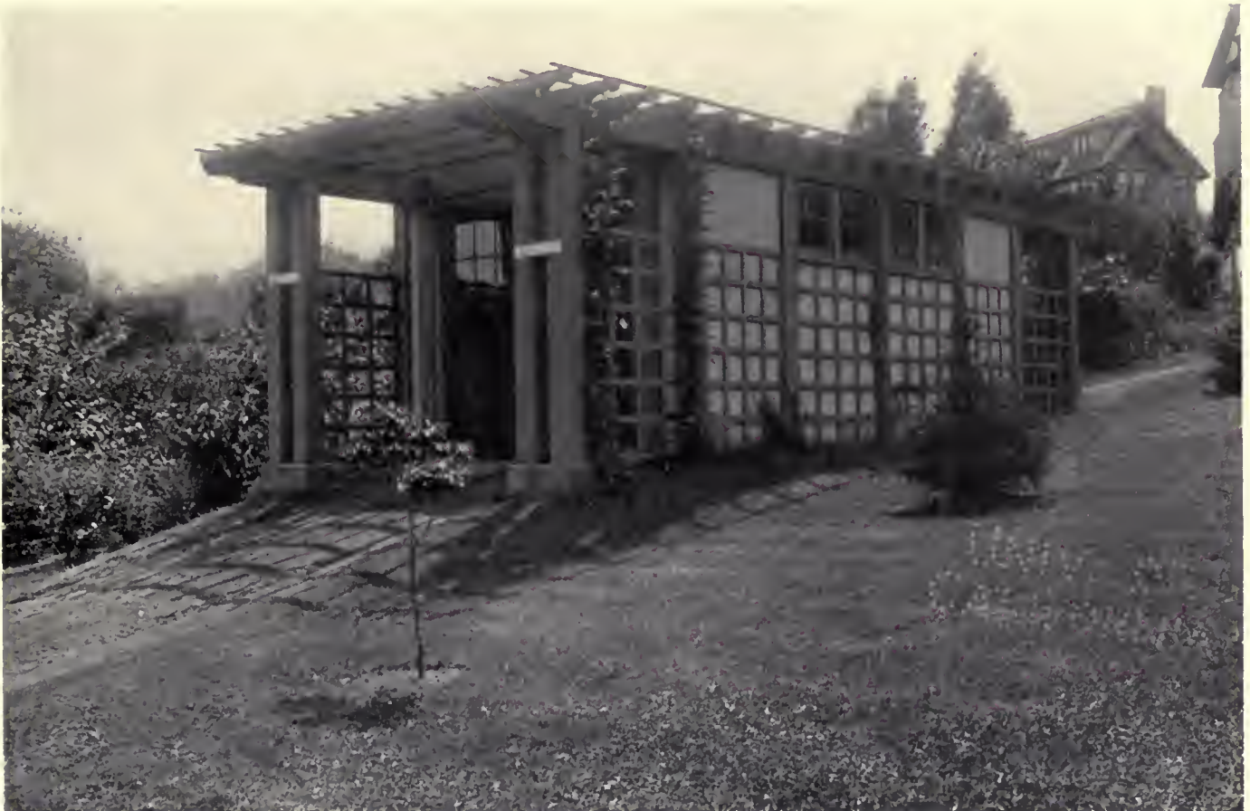
A CEMENT GARAGE WITH PERGOLA, AT MONTCLAIR, N. J. This garage is built on a hillside corner lot. Road runs through the building, so that car may enter at one end and leave at the other
