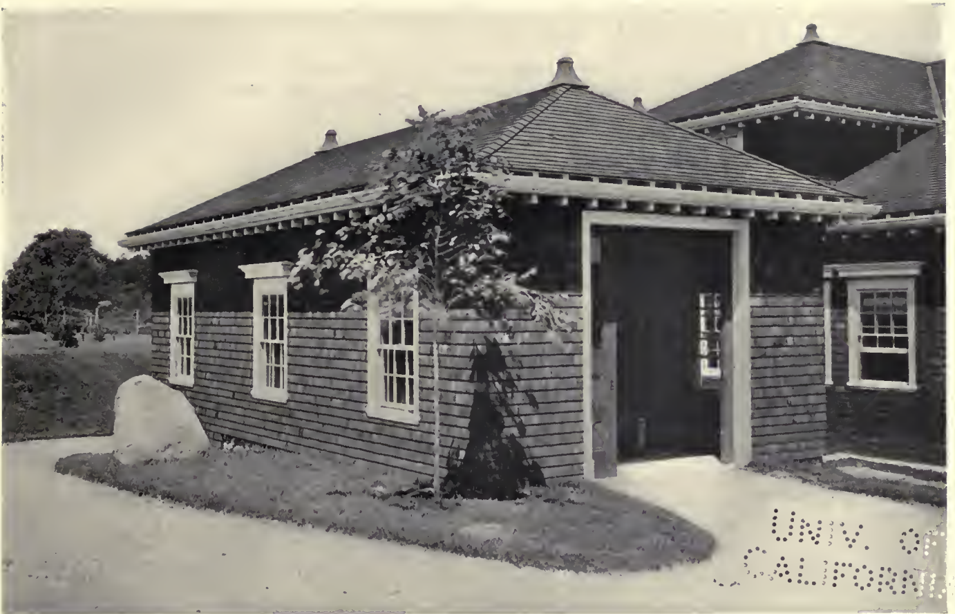
ONE-CAR GARAGE AT NEWPORT, R. I. Edward P. Whitman, Architect
