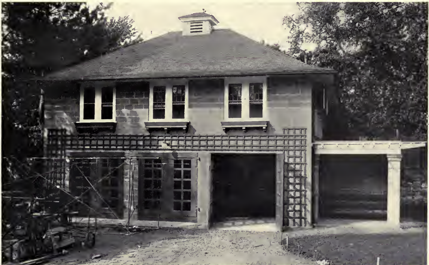
A GARAGE BUILT OF CONCRETE BLOCKS AT ENGLEWOOD, N. J. Davis, McGrath & Kiessling, Architects
