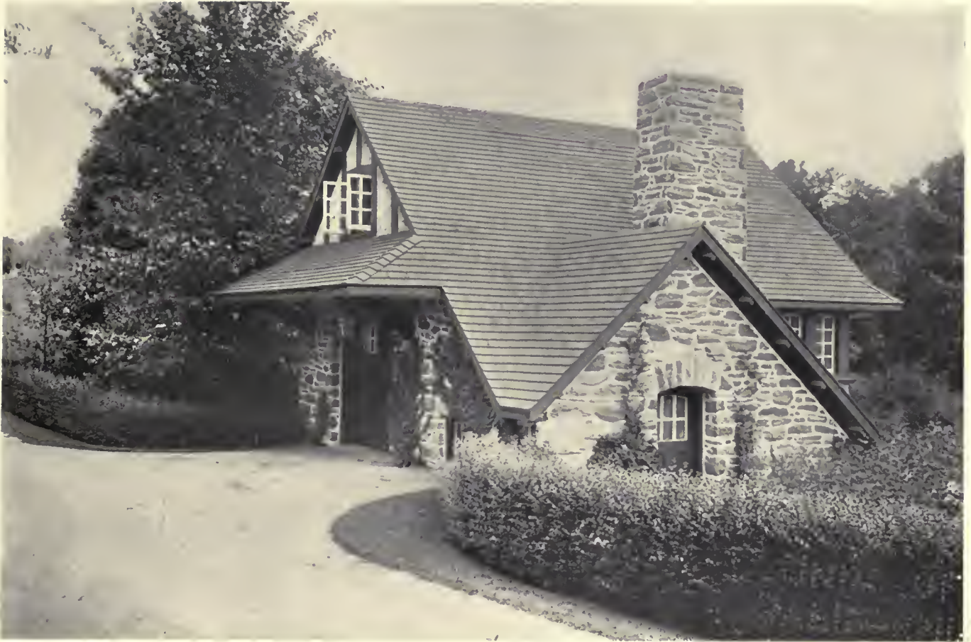
GARAGE AT ROSEMONT, PA. Built of local stone, with shingle roof
