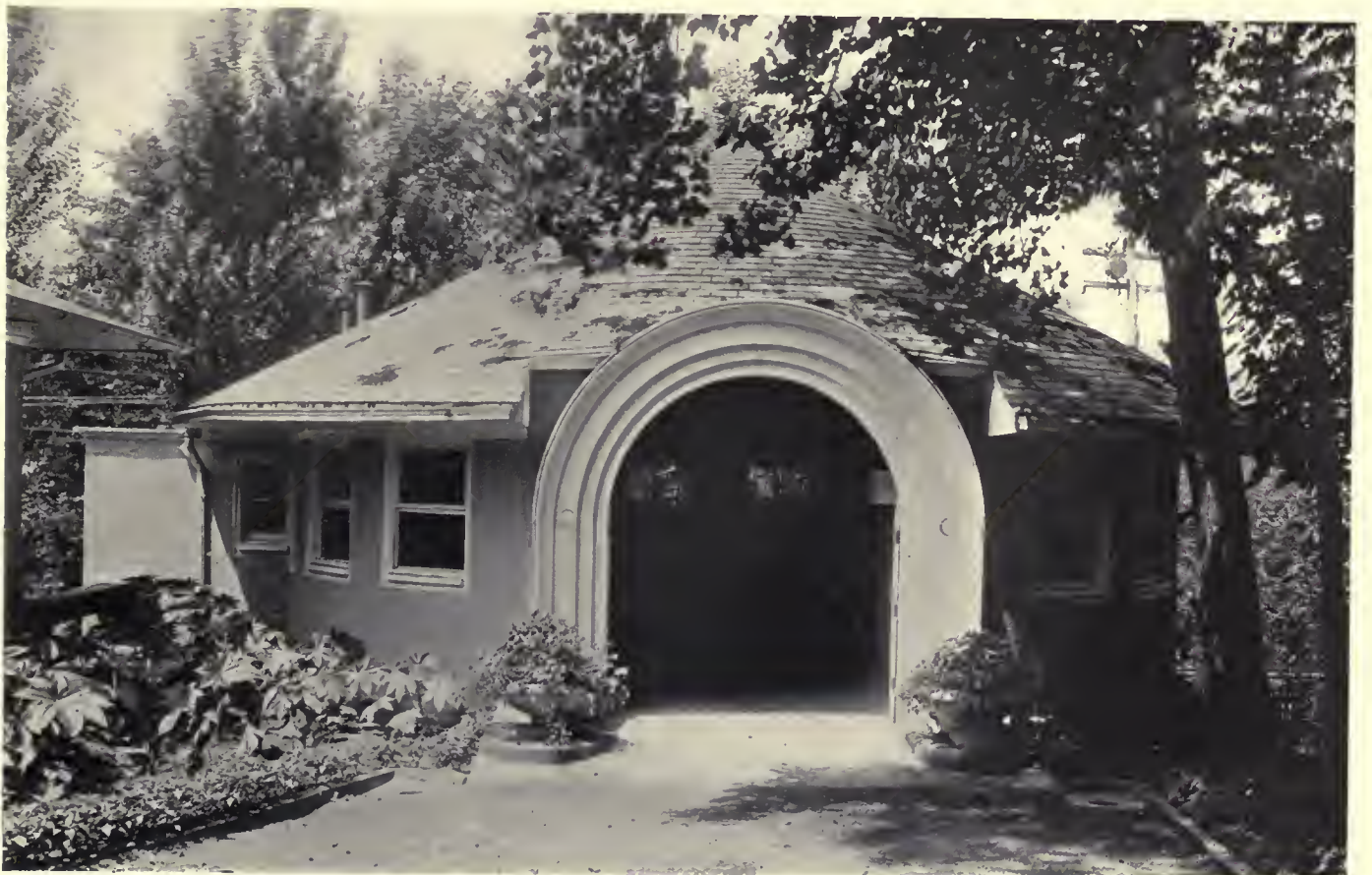
A CIRCULAR GARAGE AT SOUTH ORANGE, N. J. George W. Maher, Architect
