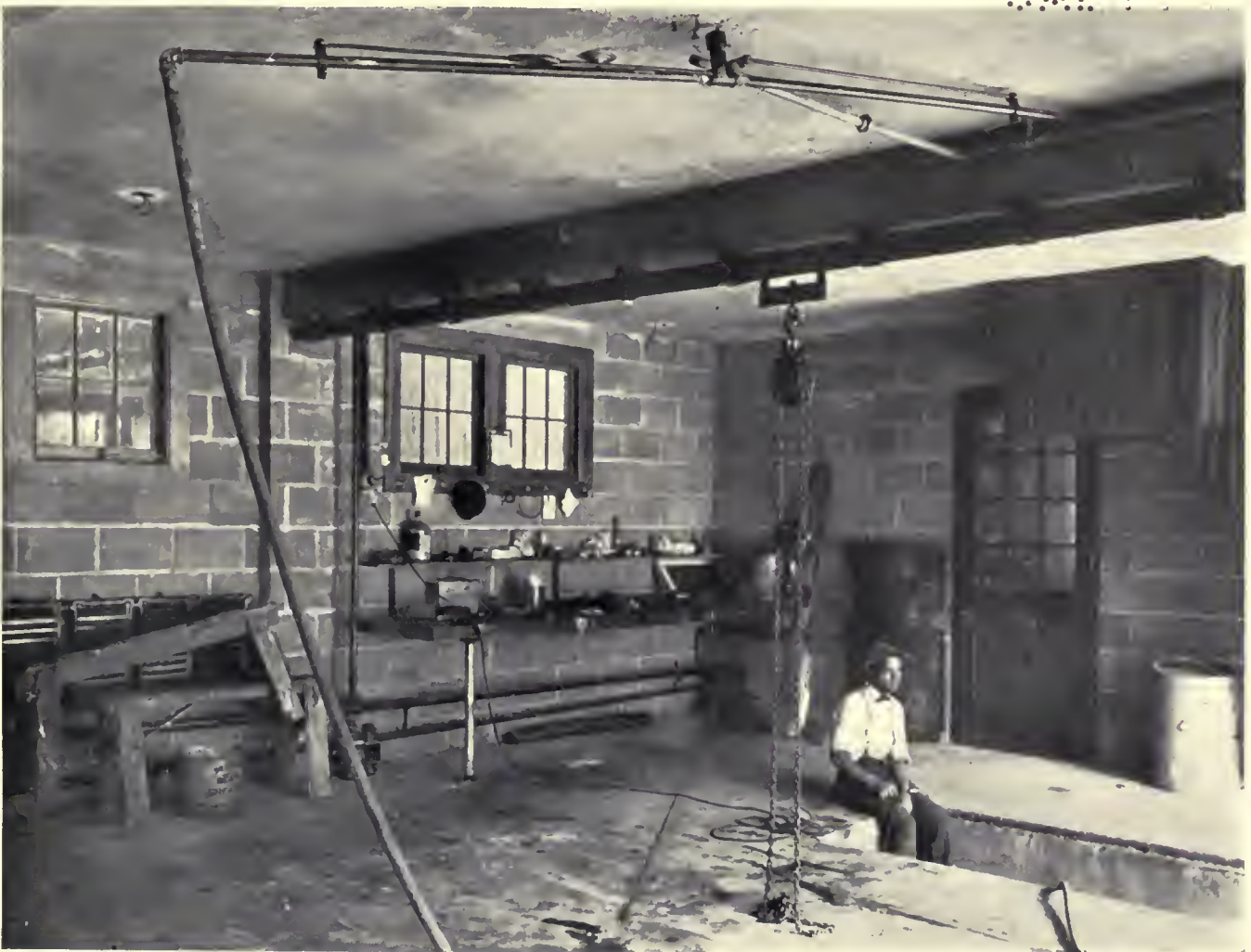
INTERIOR OF GARAGE AT ENGLEWOOD, N. J., SHOWING WORKBENCH, PIT, OVERHEAD WASHER AND TRAVELING HOIST Messrs. Davis, McGrath & Kiessling, Architects
