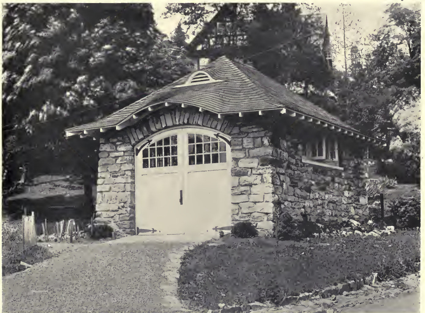
GARAGE OF FIELD STONE WITH SHINGLE ROOF AT LAWRENCE PARK, BRONXVILLE, N. Y.
