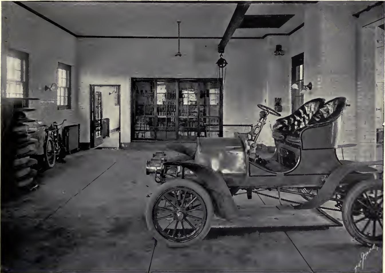
INTERIOR VIEWS OF GARAGE AND POWER HOUSE AT TOPSFIELD, MASS. Putnam & Cox, Architects
