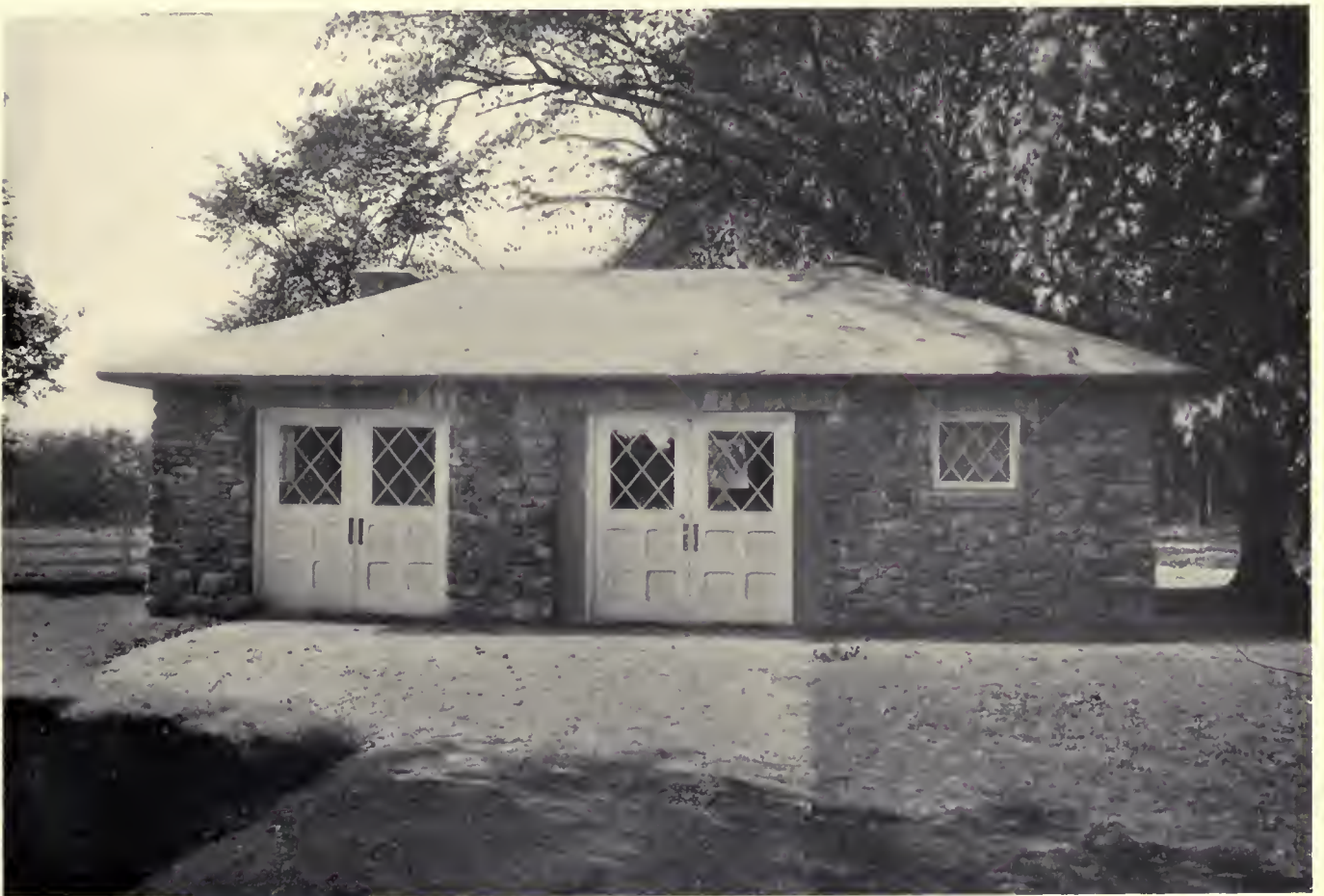
A GARAGE AT "GRASSLANDS," EAST VIEW, N. Y. Built of field stone with concrete roof
