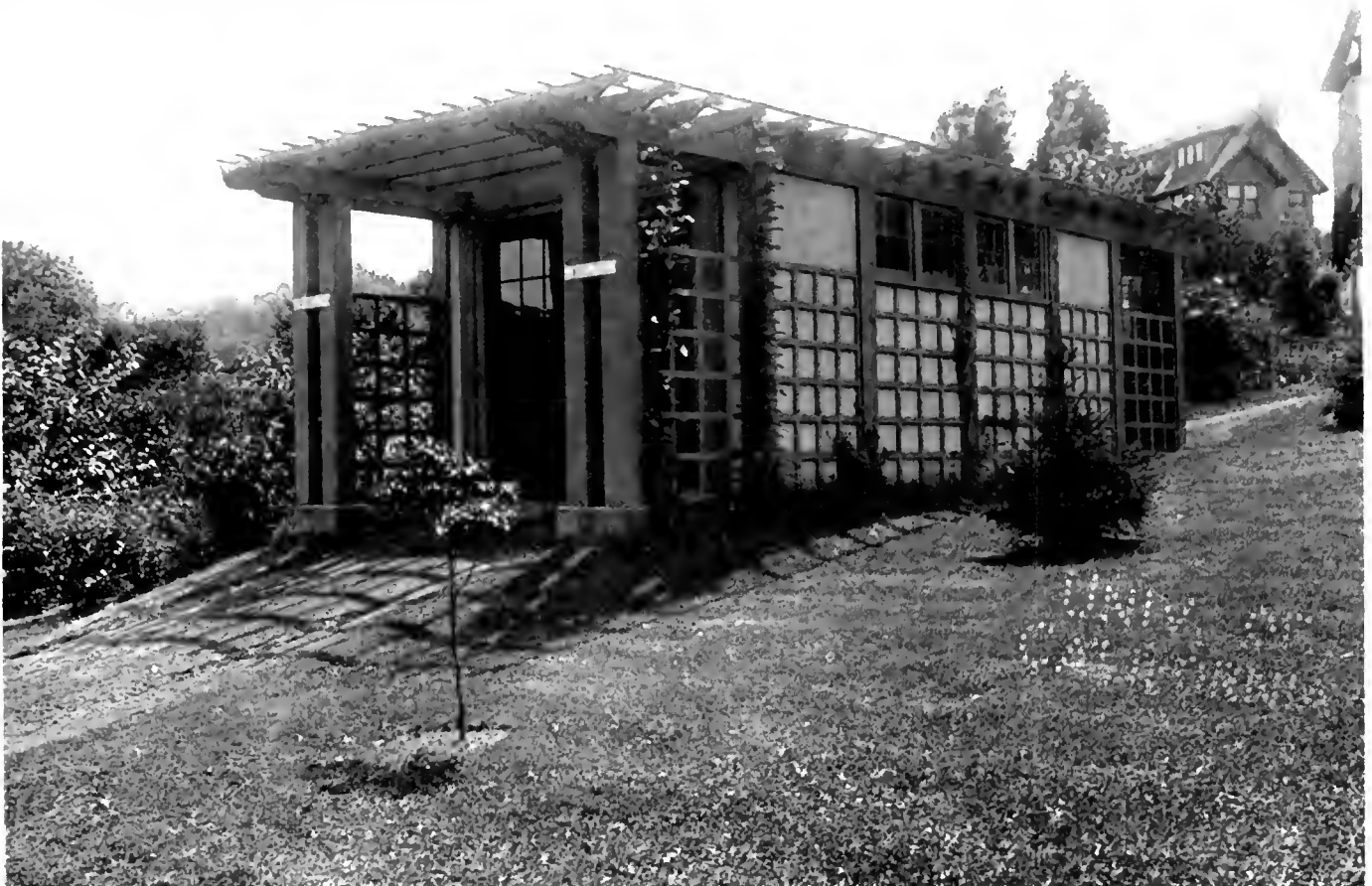
A CEMENT GARAGE WITH PERGOLA, AT MONTCLAIR, N. J. This garage is built on a hillside corner lot. Road runs through the building, so that car may enter at one end and leave at the other
