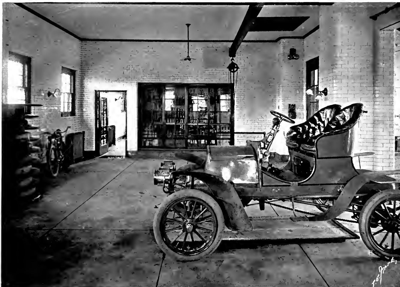
INTERIOR VIEWS OF GARAGE AND POWER HOUSE AT TOPSFIELD, MASS. Putnam & Cox, Architects
