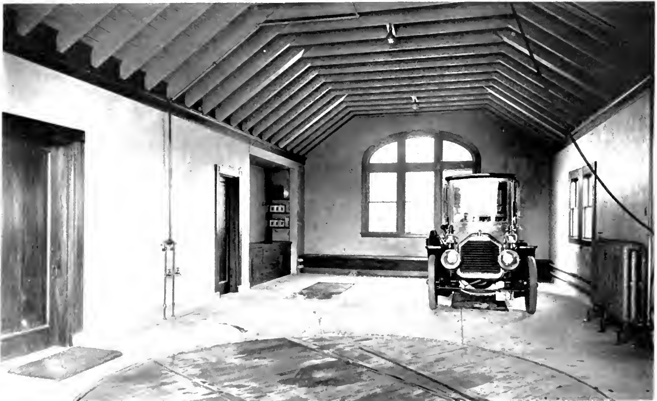
INTERIOR OF A GARAGE AT BROOKLINE, MASS., SHOWING TURNTABLE Putnam & Cox, Architects
