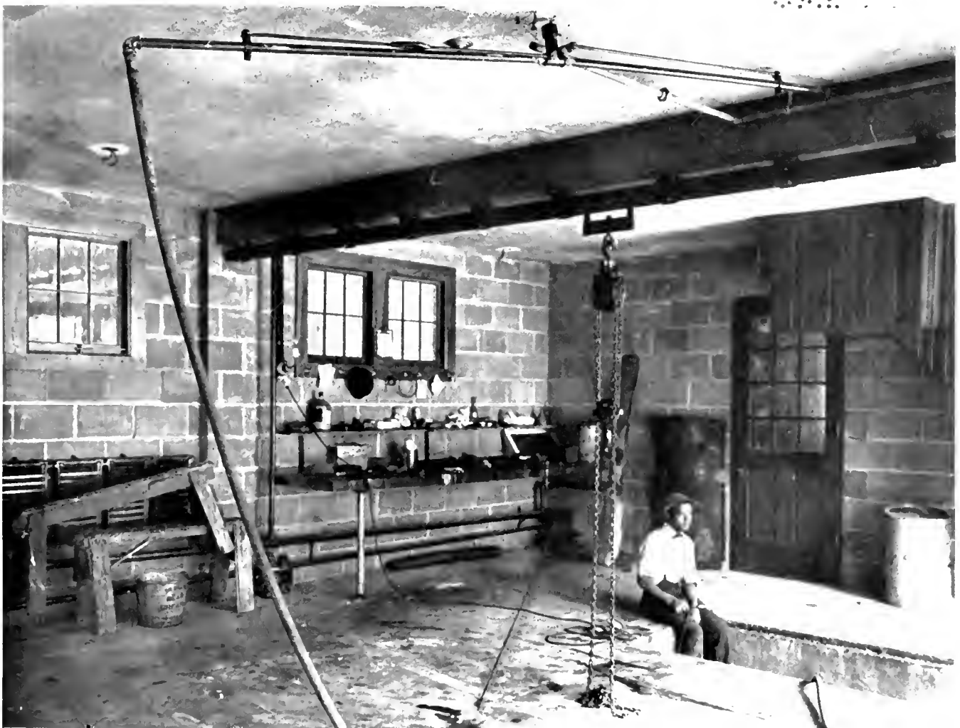
INTERIOR OF GARAGE AT ENGLEWOOD, N. J., SHOWING WORKBENCH, PIT, OVERHEAD WASHER AND TRAVELING HOIST
