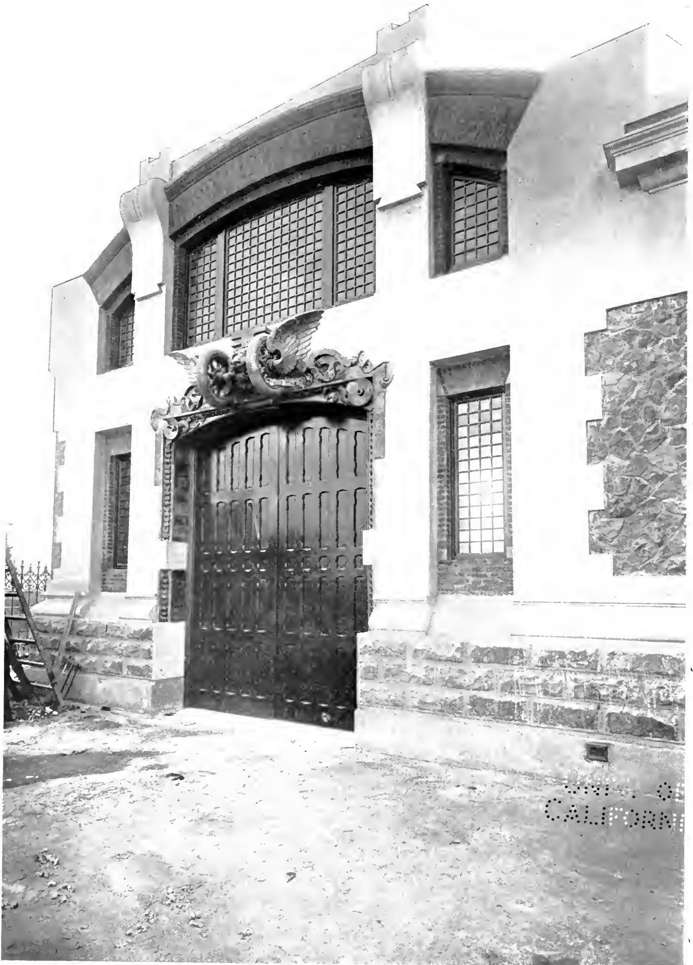
GARAGE OF CHARLES BEYERLE, ESQ., CAIRO, EGYPT Carlo Prampolini, Architect
