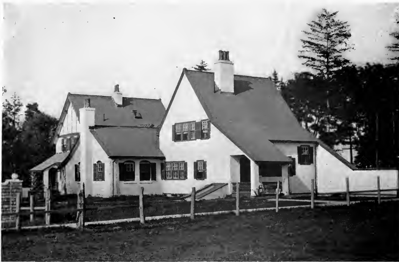
REAR OF GARAGE AT BRISTOL, R. I.
