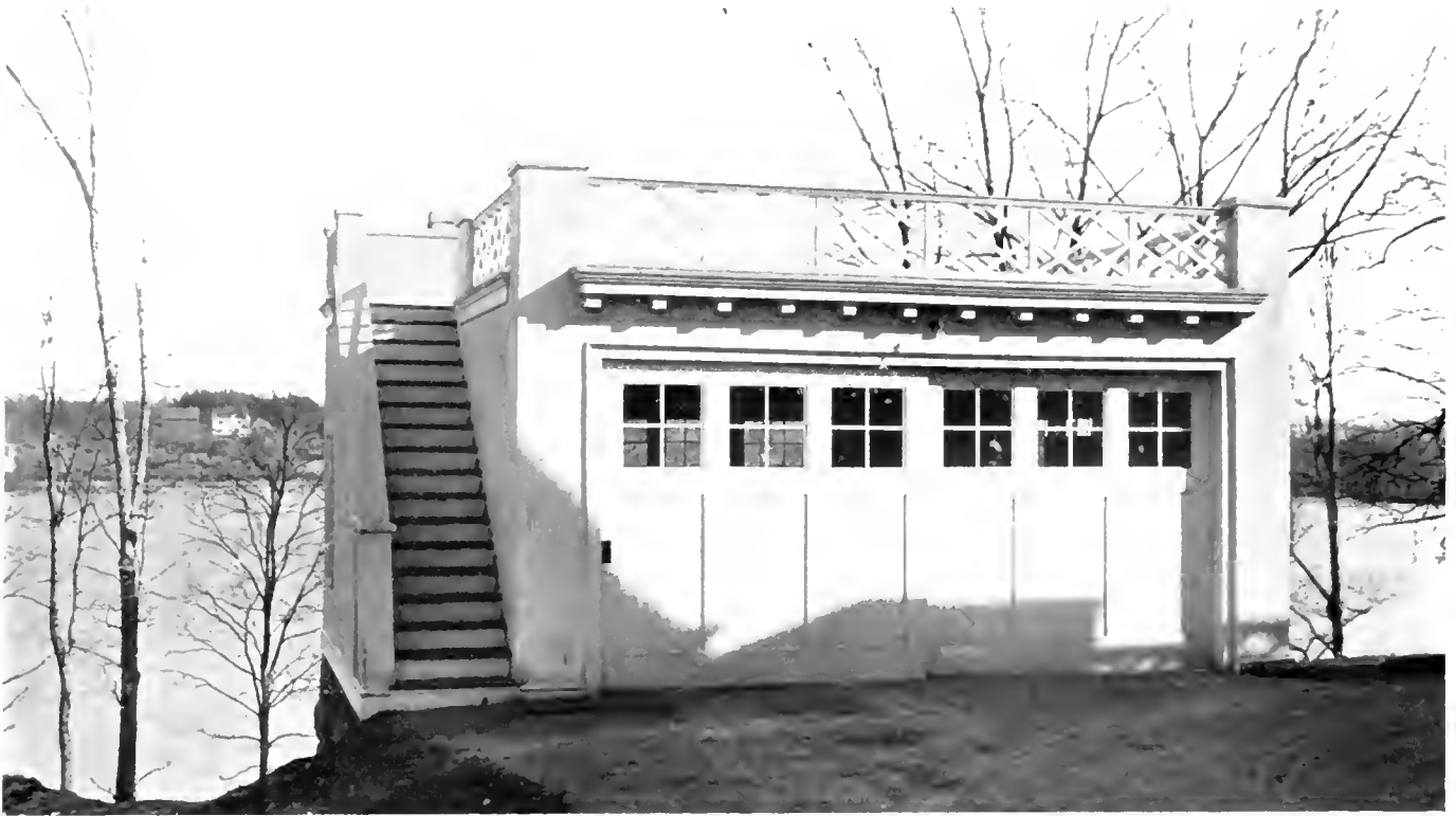
CONCRETE GARAGE OVERLOOKING LAKE NEAR WINCHESTER, MASS.
