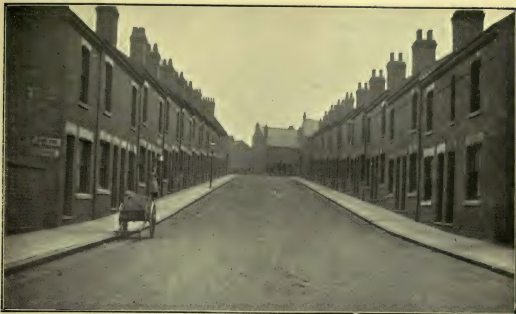
A typical new street of an industrial town. The houses are built forty or more to the acre, and in this instance the frontages are 12 feet only.
