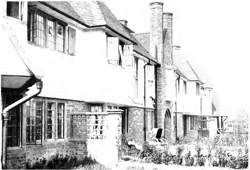
FOUR HOUSES AT SOUTH VIEW
