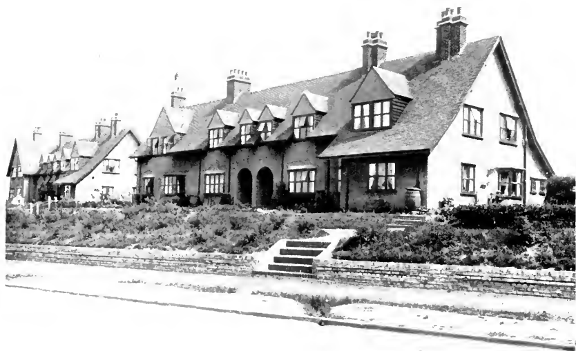
WORKMEN'S COTTAGES AT RIDGE ROAD (GARDEN CITY TENANTS, LTD.)
