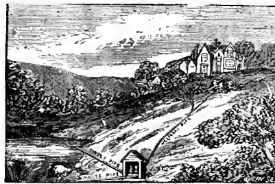
View of Ram worked by Water from a spring, and supplying the house and garden on the hill.
