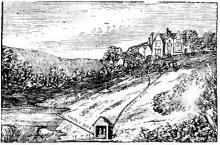
View of Ram worked by Water from a spring, and supplying the house and garden on the hil'.
