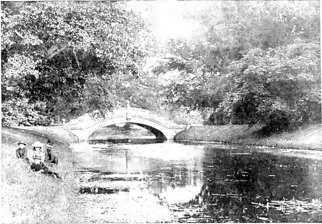
FIG. 123.—CHINESE BRIDGE IN THE PLEASURE-GROUNDS, WREST PARK. (SEE P. 374.)
