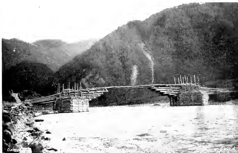
FIG. 82.—BRIDGE OVER TOW RIVER.
