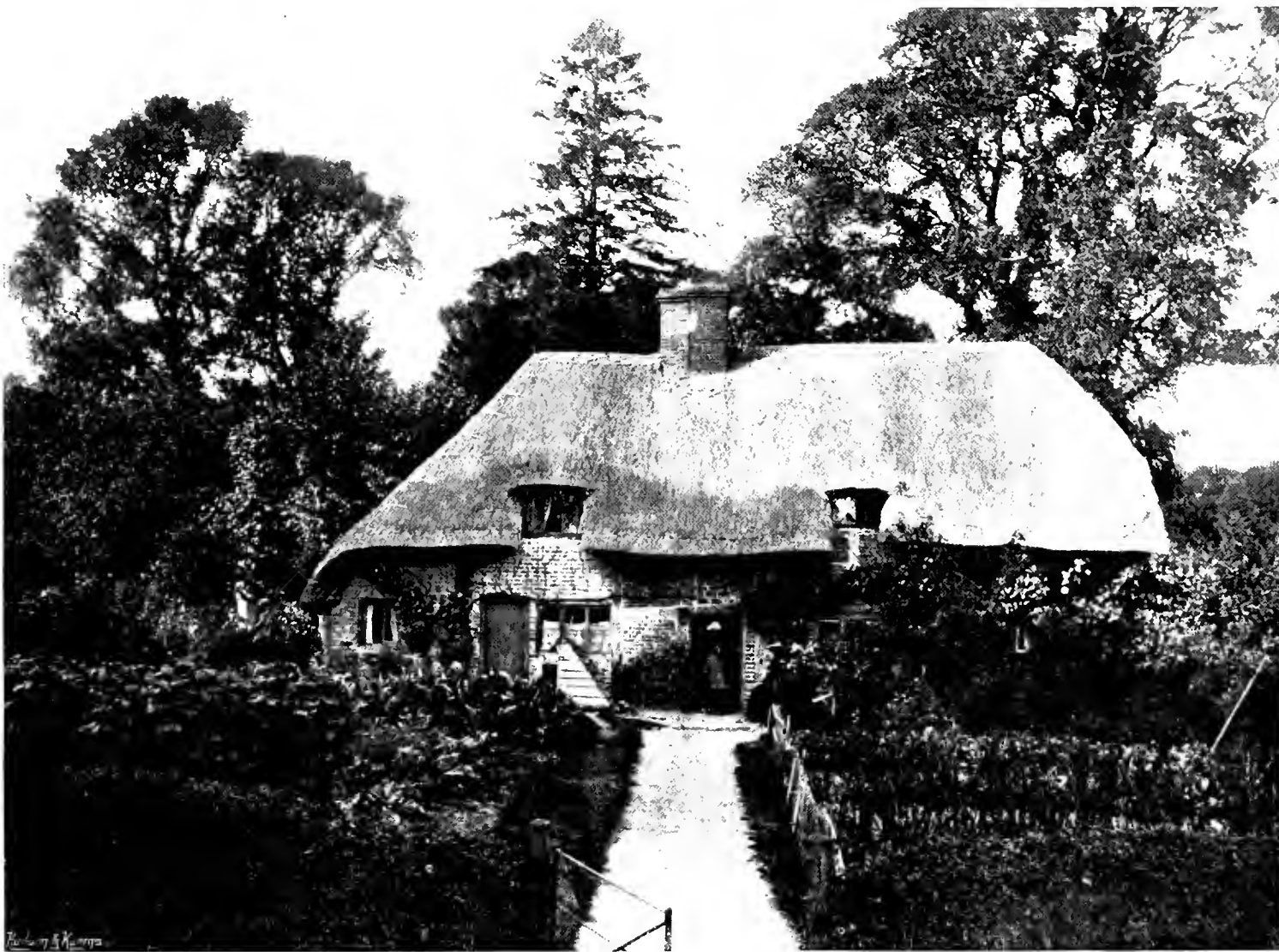
A COTTAGE AND GARDEN AT DEANE, NEAR BASINGSTOKE.
