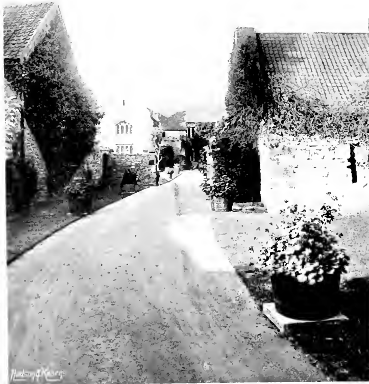
MATHERN PALACE. THE ENTRANCE THROUGH THE RUINED GATEWAY.
